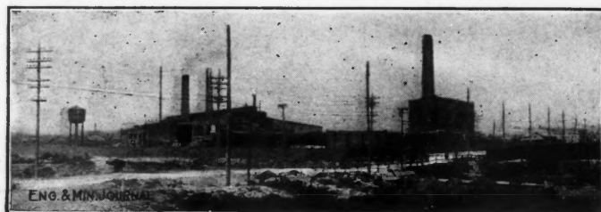
INTERNATIONAL LEAD REFINING Co.'s PLANT, EAST CHICAGO, IND. Flue in foreground, baghouse at right.
