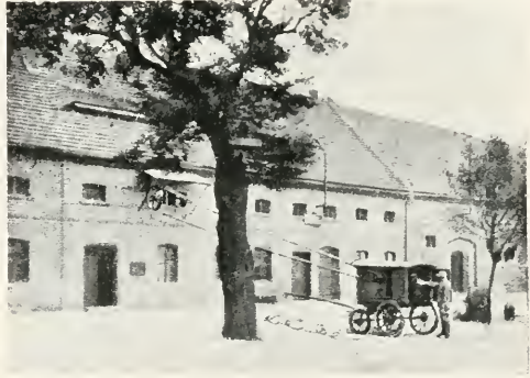
Portable Motor connected with Chaff-cutter in a left on a German farm.—Illustration by Siemens Bros., Ltd.
