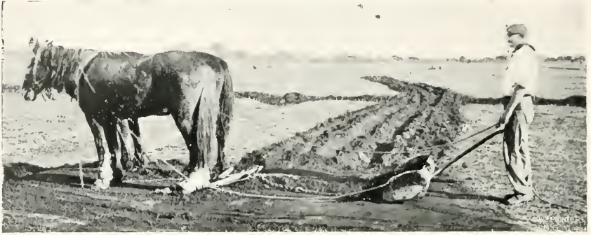
Contractor working buck-scraper.
