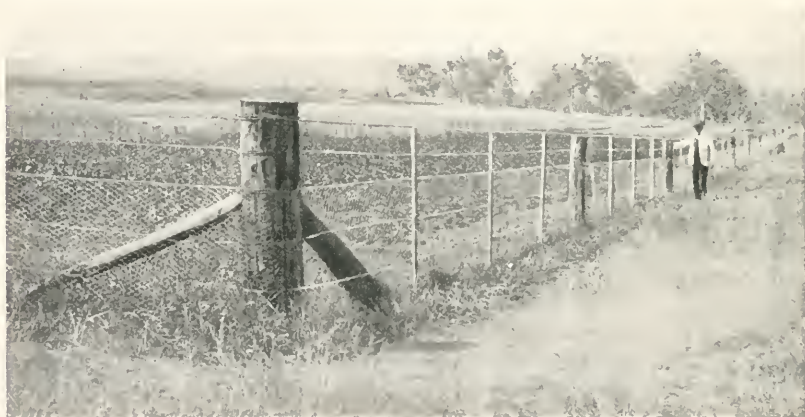
A wire-netted rabbit-proof fence, two posts and six droppers per chain.
