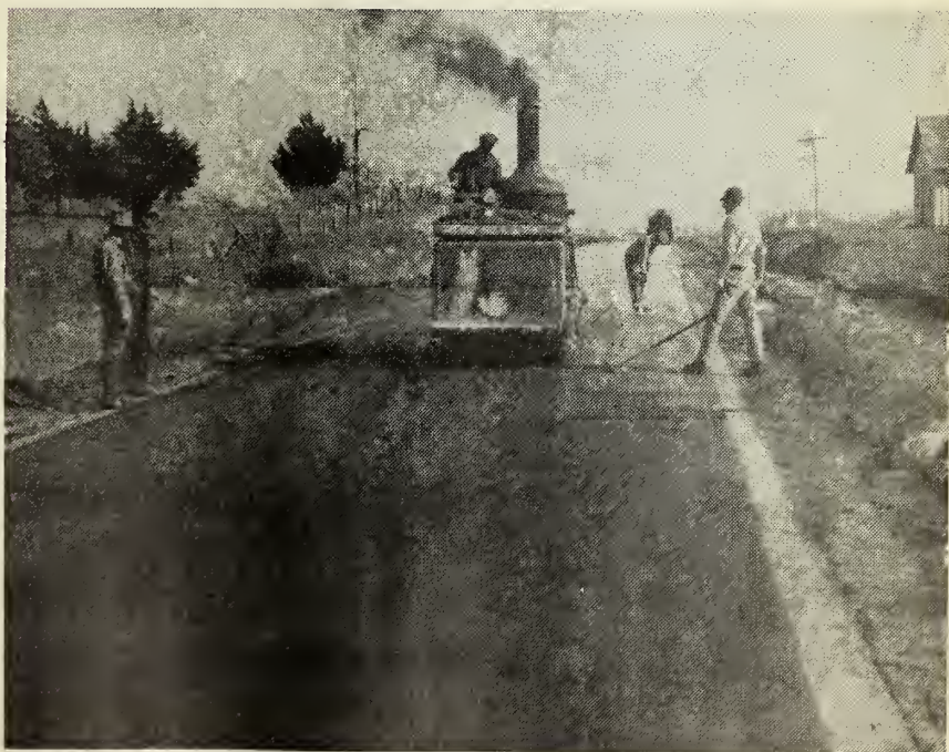
Fig. 4. - The surface was completely sealed by the roller
