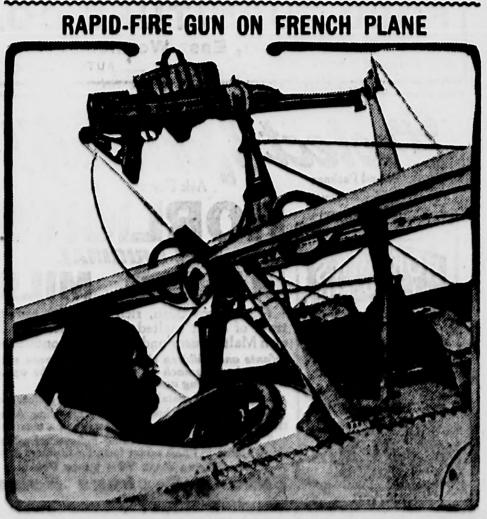
The little French Nieuport "scout" plane is the greatest fighting machine airmen, who has brought down his and is equipped with an electric rapid-fire gun which is worked from the pilot seat by a wire.
