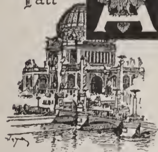
The Administration Building
