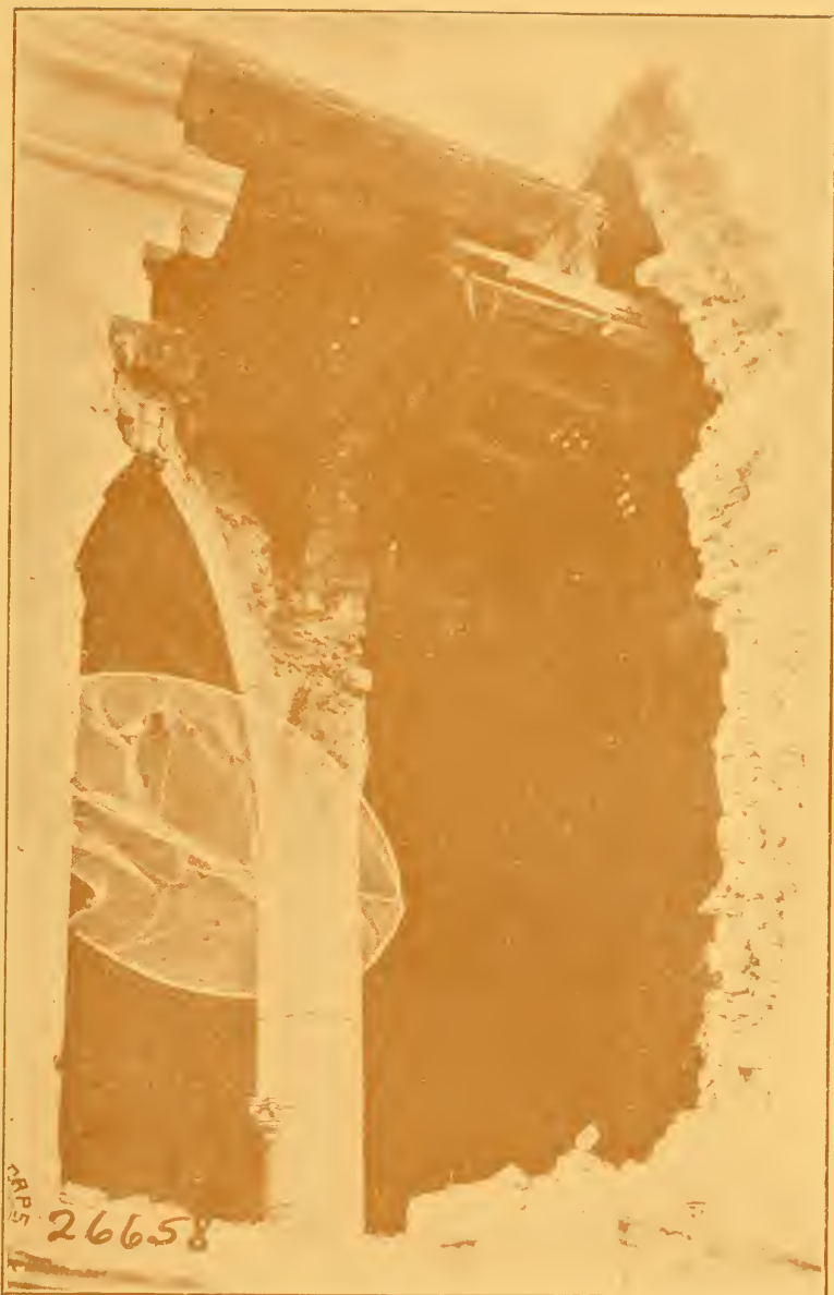
Hole in wall of church in Grandpre caused by one German shell. Headquarters Co. "E" in church at the time the shell struck.
