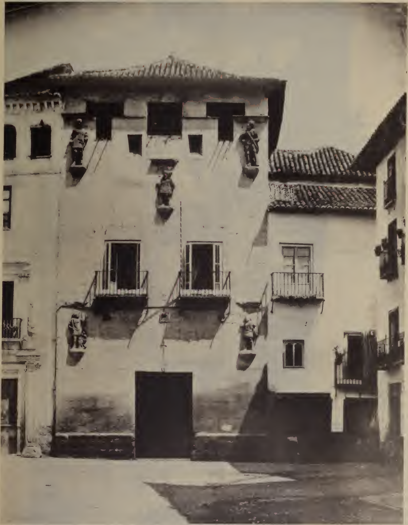
GRANADA—HOUSE OF THE TROS
