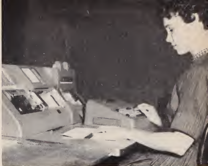
At the center, data sheets are translated into punches on a card in preparation for the high-speed totaling.
