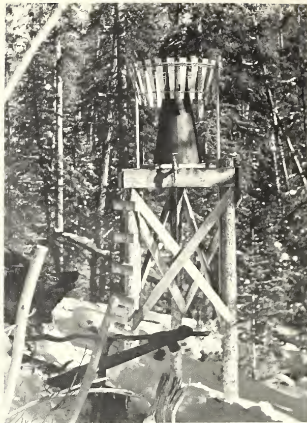
Figure 122. Sacramento-type seasonal storage gage at the Iron Creek site. November 1946.
