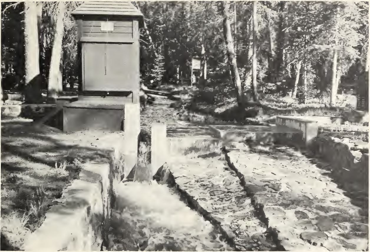
Figure 127. Looking upstream at Fool Creek gaging station, June 1949.
