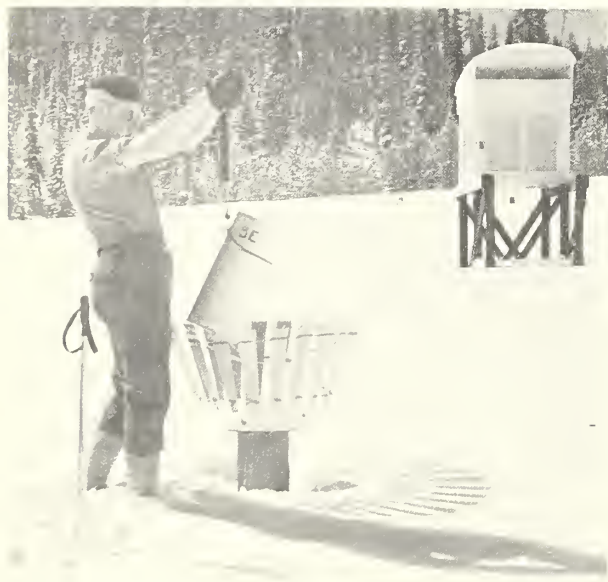
Figure 124. Weighing an 8-inch precipitation gage at West St. Louis Station, April 1950.
