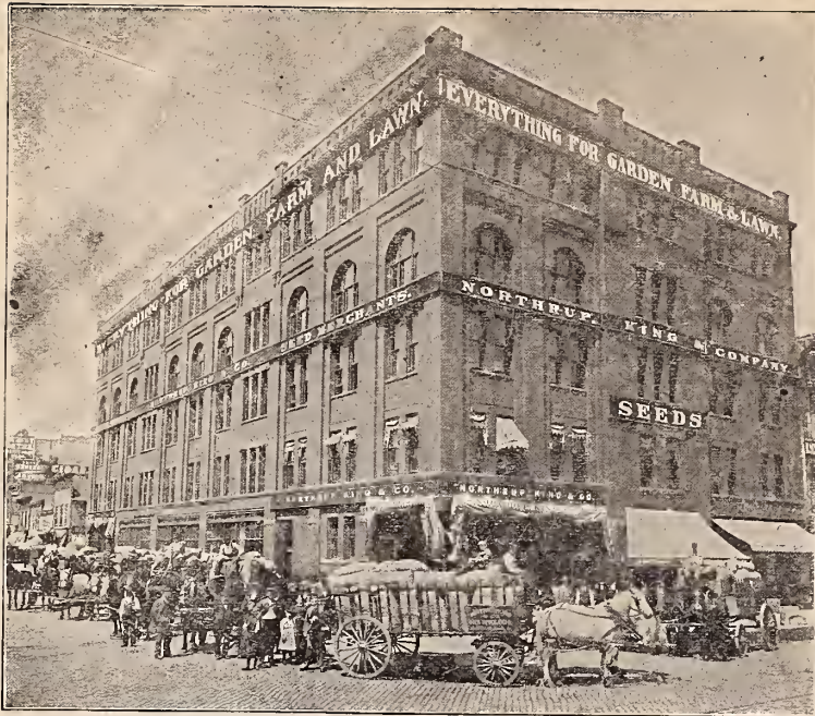
OUR SEED WAREHOUSE. "LOADING OUT FOR THE DEPOTS." FROM A PHOTOGRAPH
