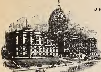
NEW STATE CAPITOL IN COURSE OF CONSTRUCTION.
