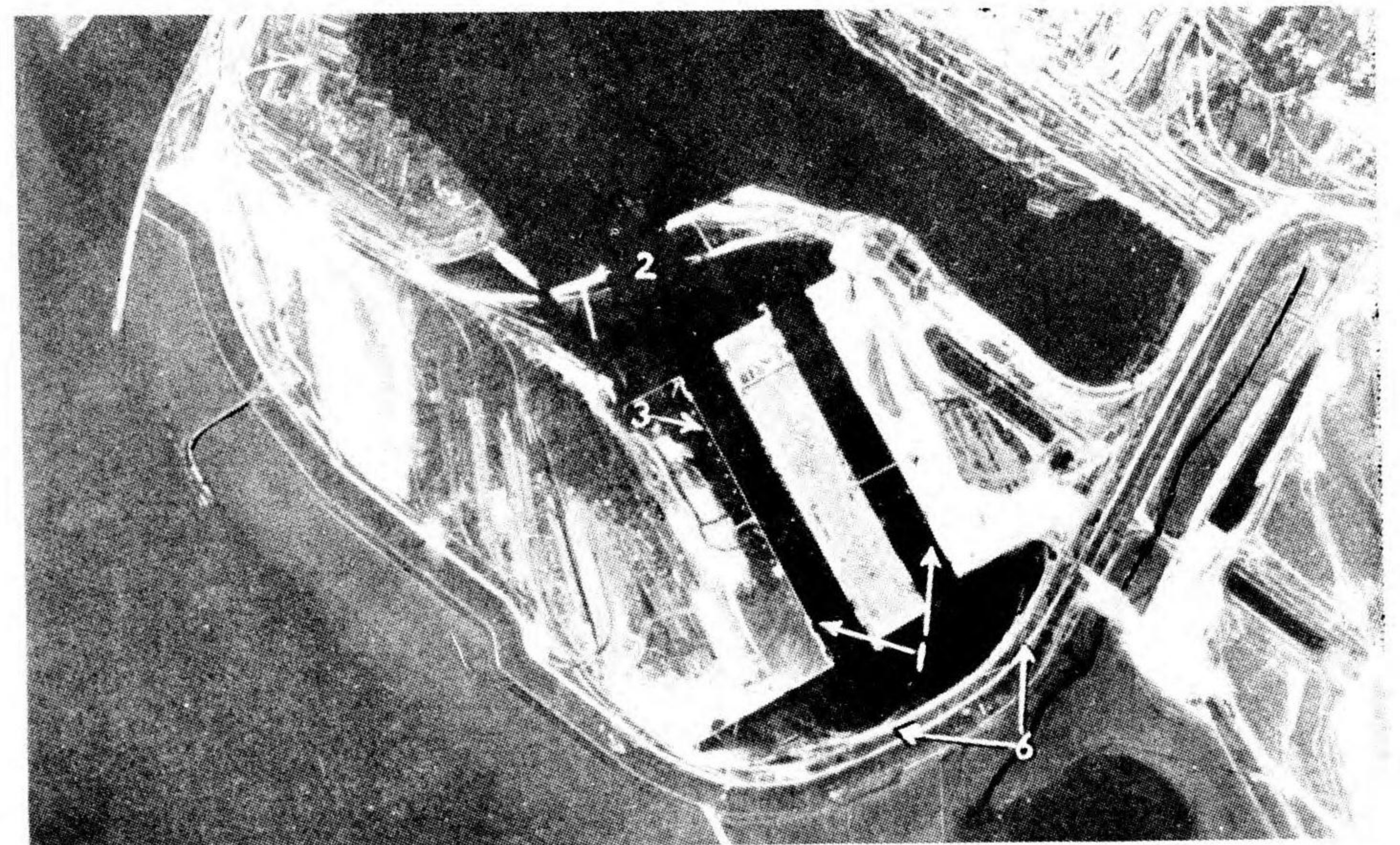
Approximate present condition. (1) new locks, 1,450 by 200 feet; (2) inner entrance; (3) completed wall of quay; (6) this wall will be removed.
