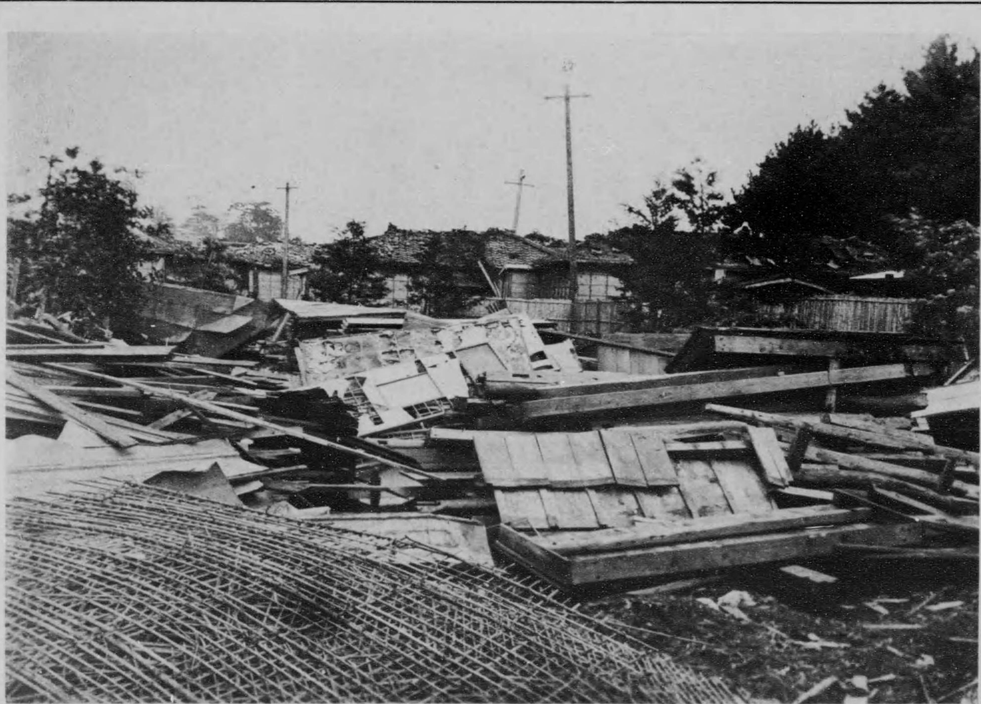
Collapsed houses at Omori, southern suburb of Tokyo.
