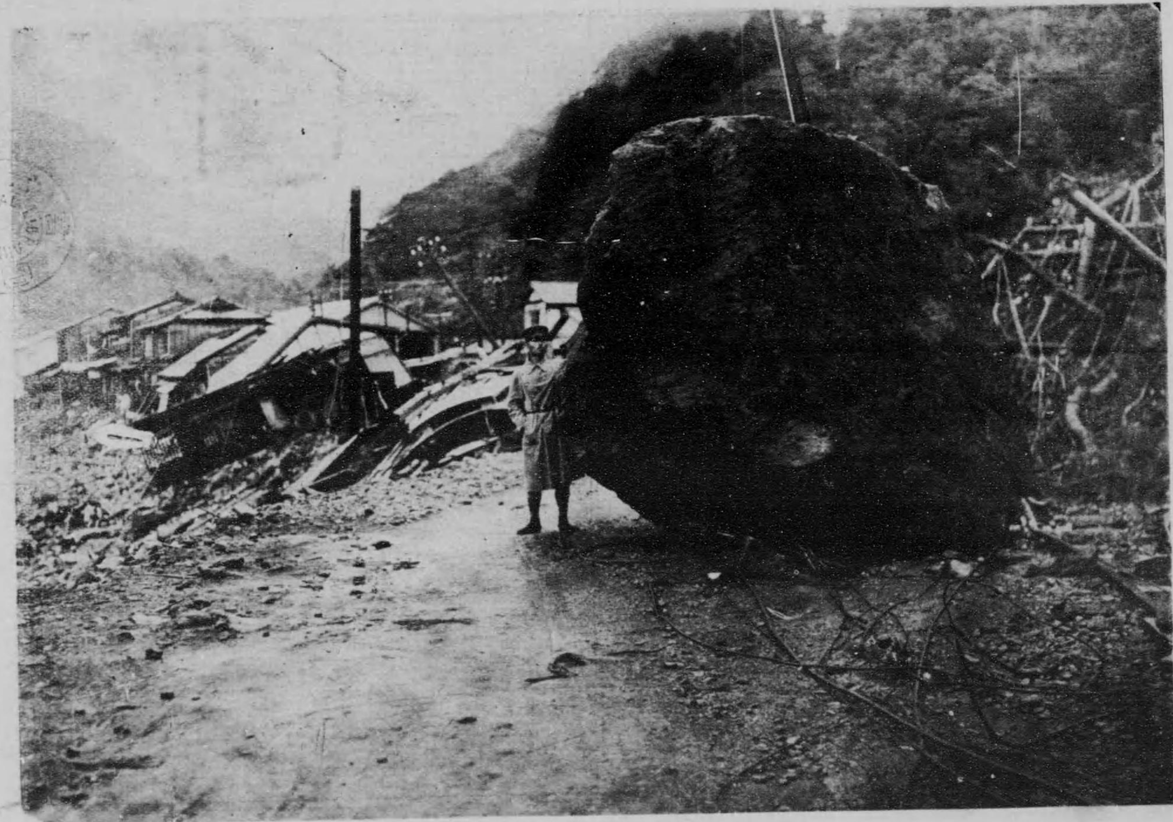
Huge stone fallen down from precipice near Yumoto Station.
