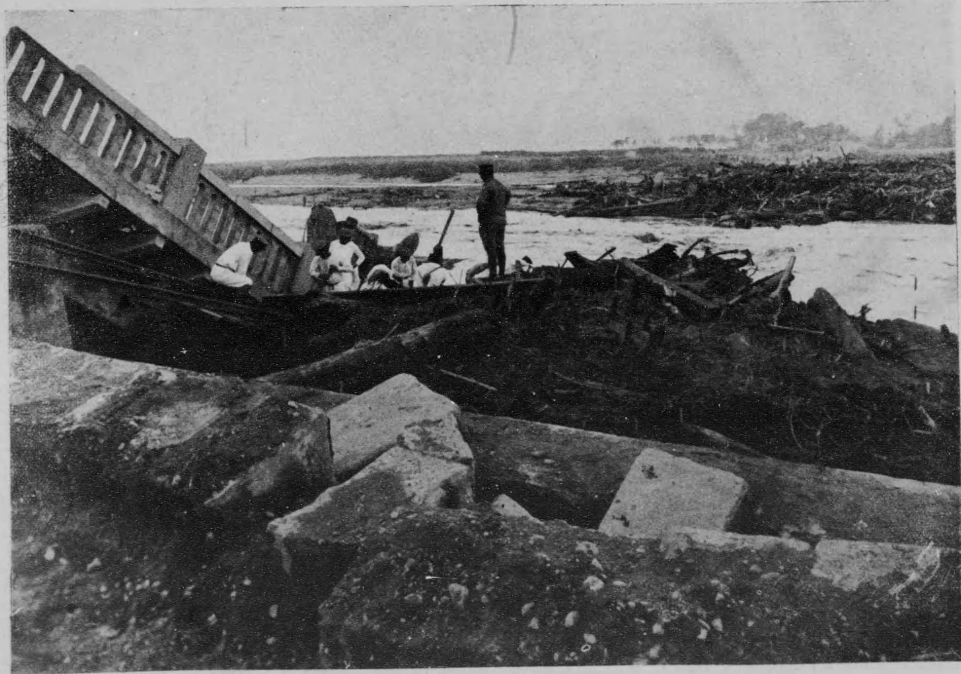
Sakawa-bashi Bridge between Odawara and Koze. The long concrete bridge lately span, was broken at the first shock.
