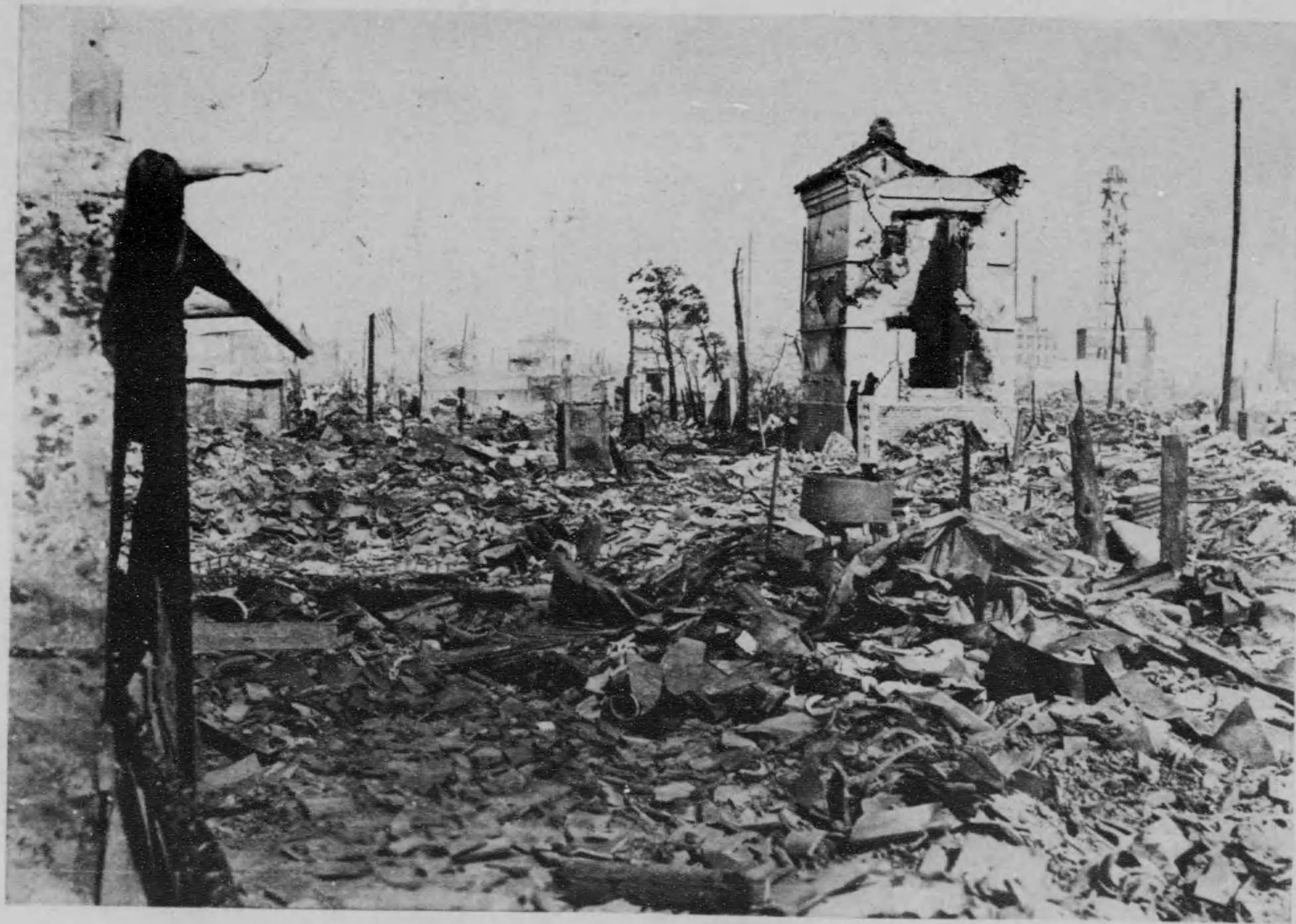
Burned ground in the vicinity of Ueno seen from Yushima, Hongo Ward.
