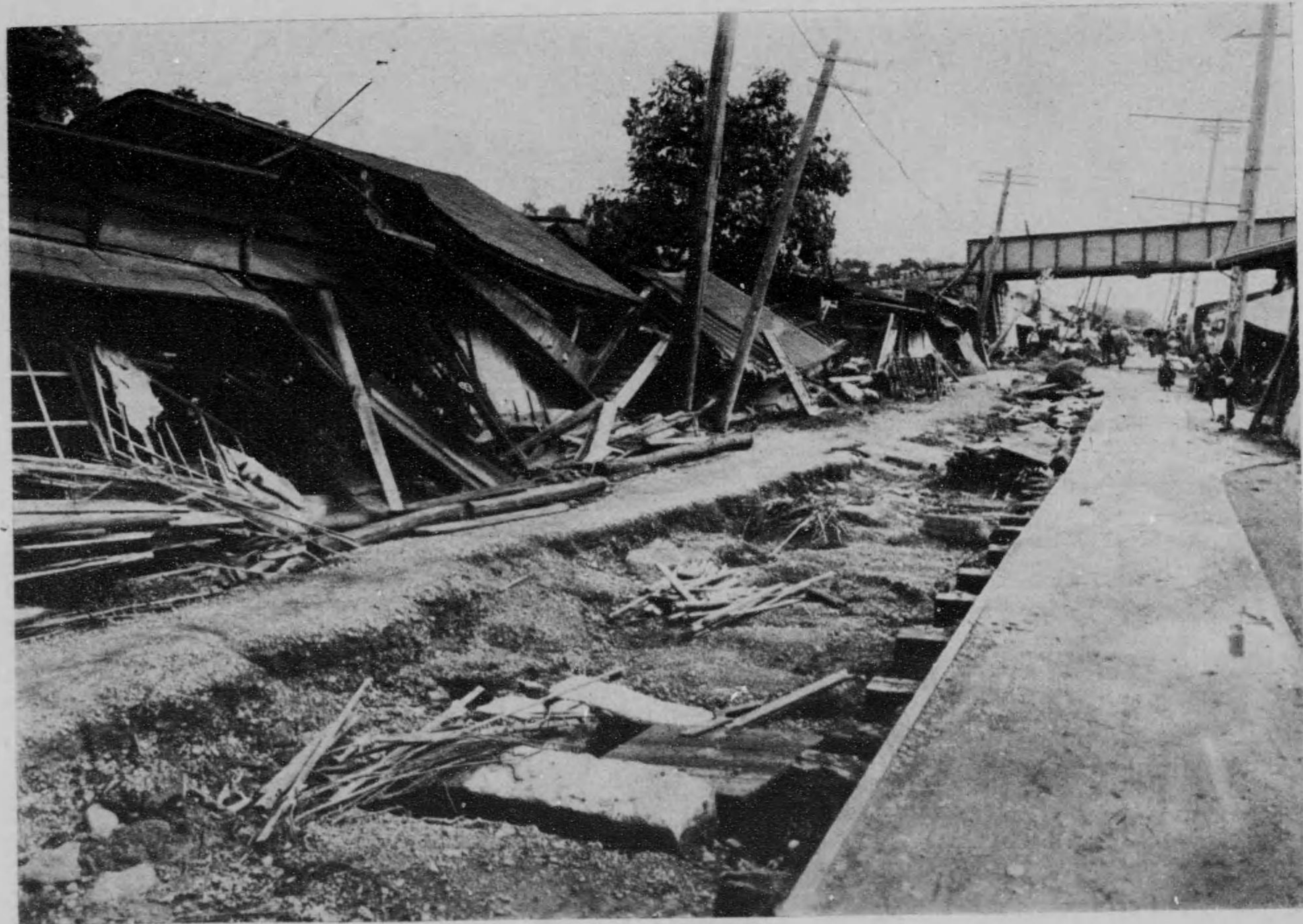
Devastation at Jujimachi, Odawara, Tokaido.
