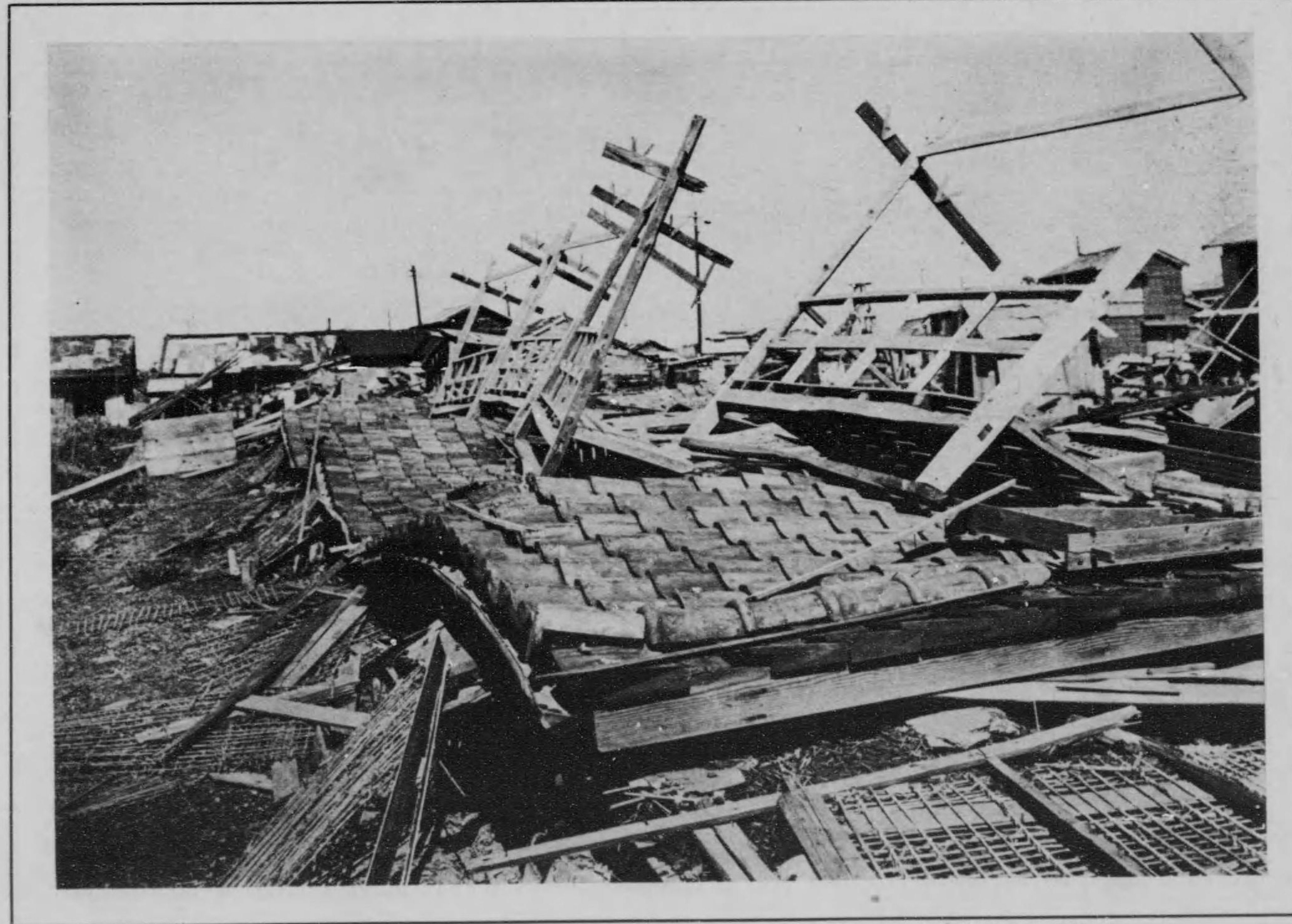
Collapsed houses at Sunamachi in eastern suburb of Tokyo. Being frail ground near the sea here, damages from shock were greater than elsewhere in Tokyo.
