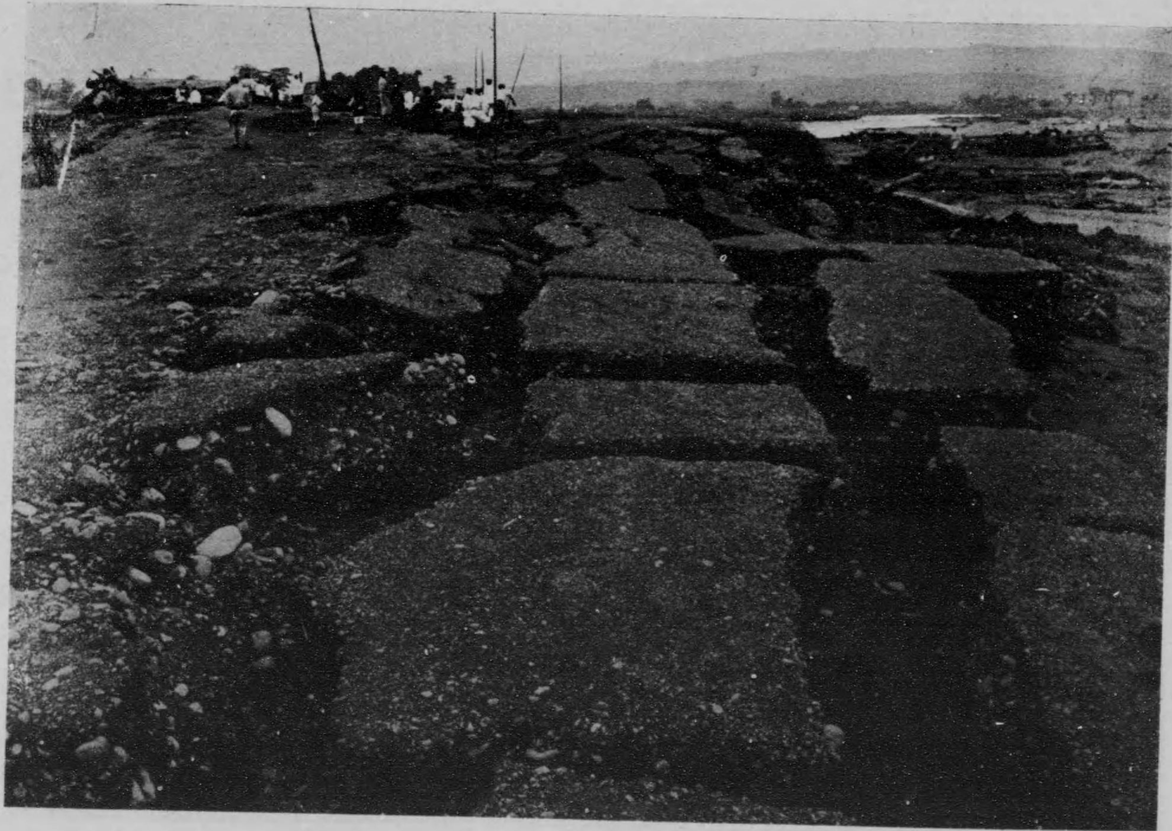
Fissures in high-way near the Sakawa River.
