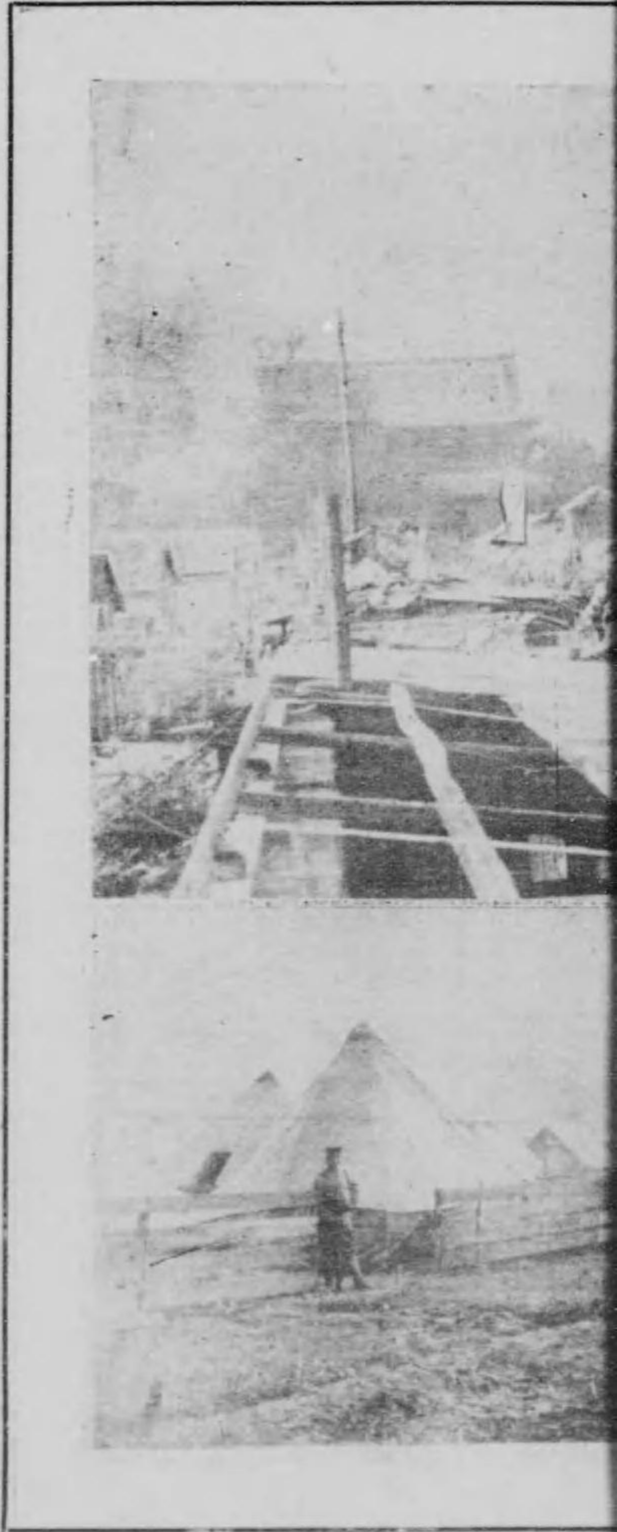
After the disaster. III. U Lower: Hospital in tents at S
