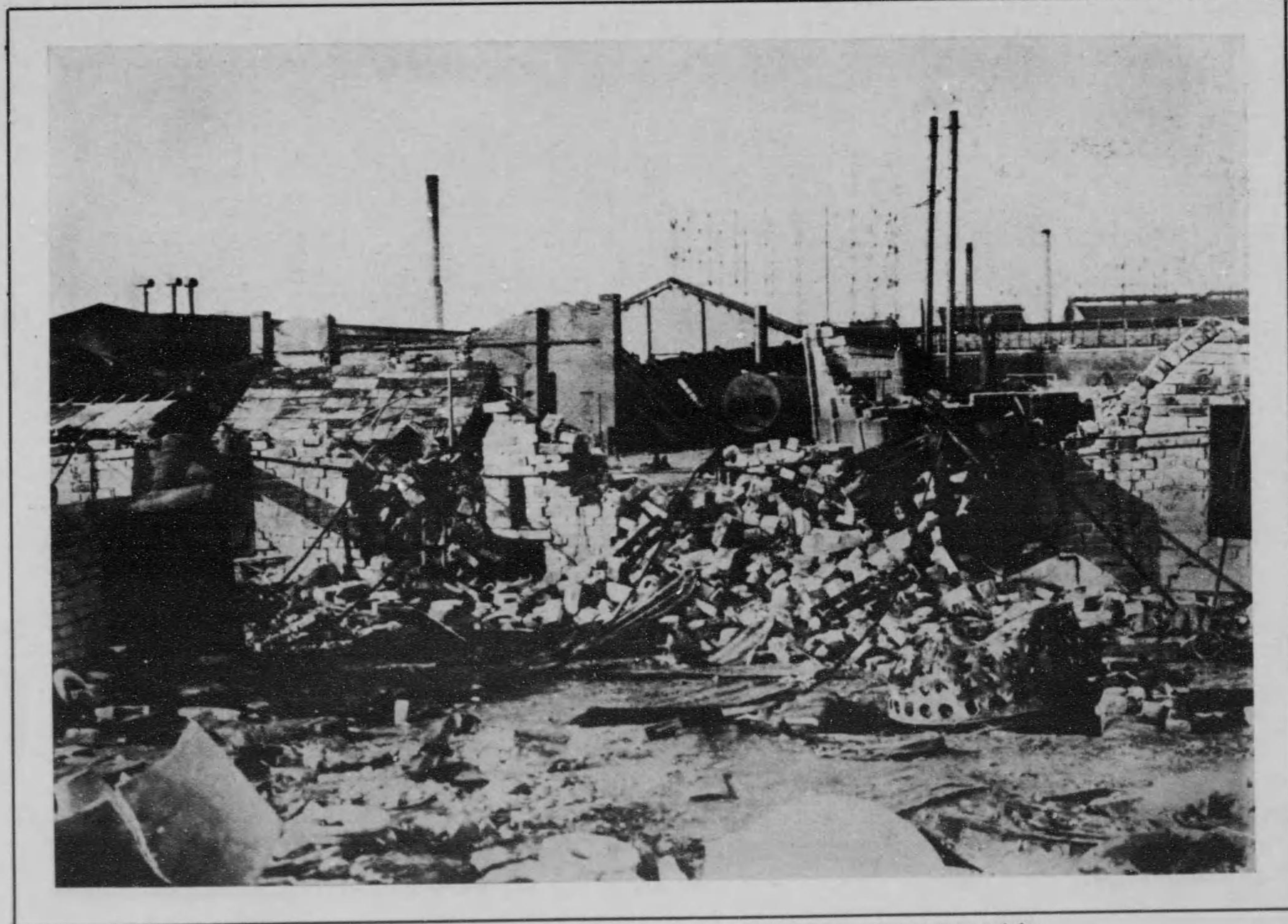
Gas-tank at Senji, Tokyo, trying to get out of the danger of explosion by evolving gas in the tank, stimulated fires on the contrary.
