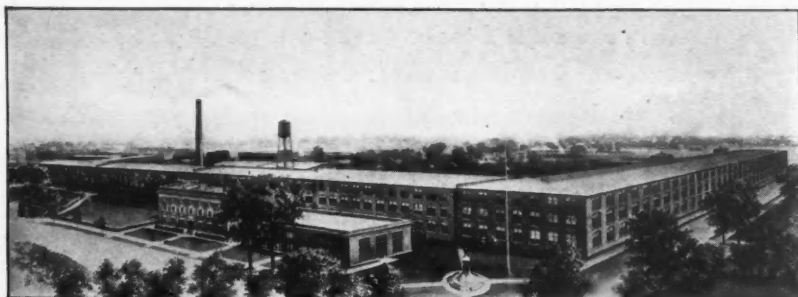
KENWOOD MILLS Albany, N. Y. Plant
