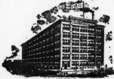
FACTORY 132 ND TO 133 RD ST & BROOK AVE
