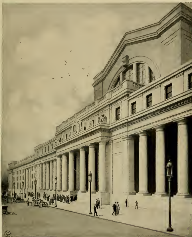
THIRTY FIRST ST. SIDE-LOOKING WEST
