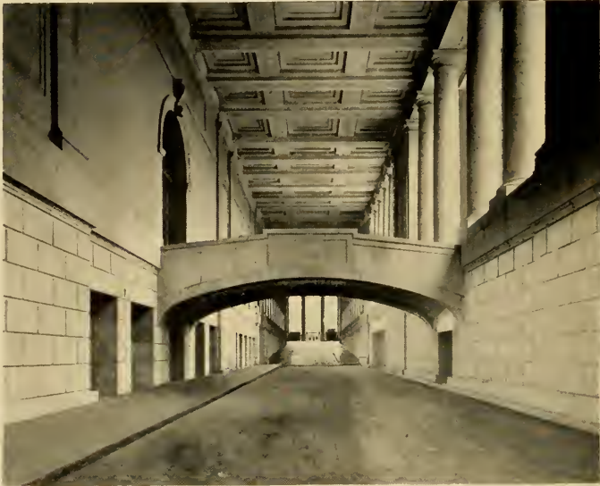
BRIDGE OVER THE DRIVEWAY
