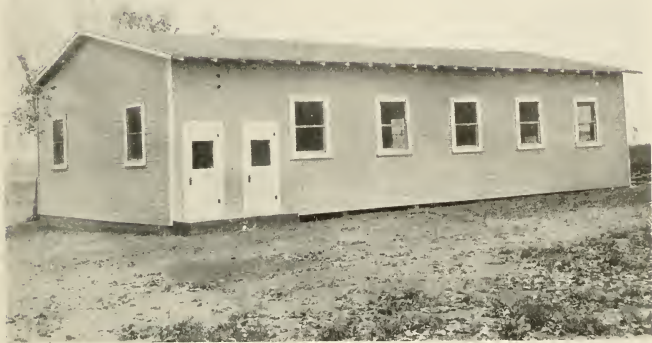
1. Shop erected at Roswell, N. Mex., in September 1930.
