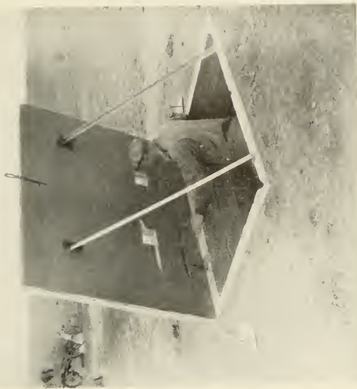
2. Concrete dugout constructed 50 feet from the launching tower so that an observer can watch the launching of the rocket at close range.
