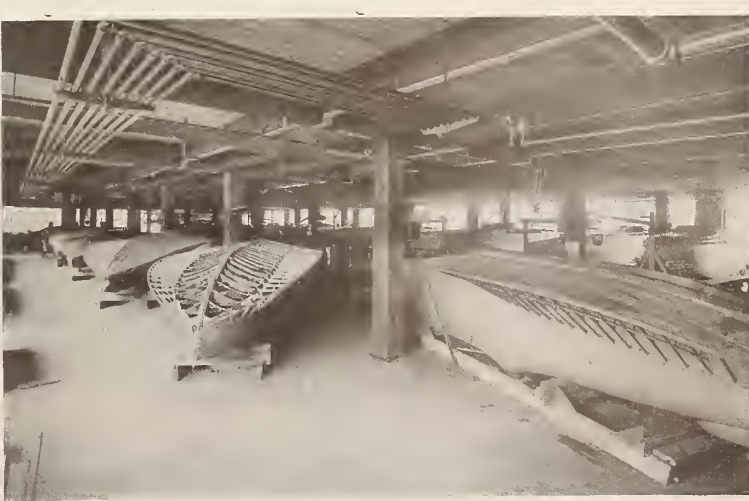
Hydro-Planes in Course of Construction at Unico Plant
