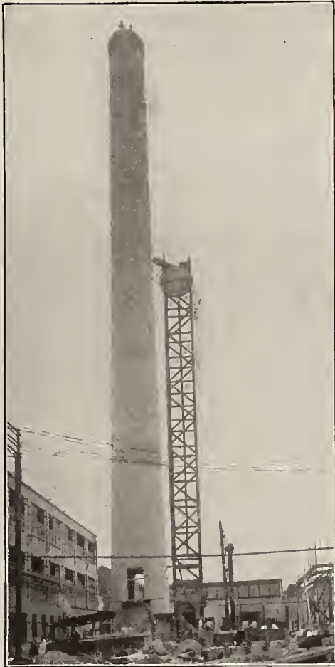
Chimney for New Edison Power House
