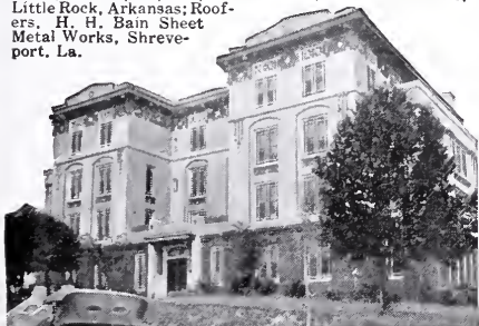
The Highland Sanitarium and Addition, Arch., C. W. King, Shreveport, La.; Gen'l Cont., Stewart-McGhee, Little Rock, Ark.; Roofers, H. H. Bain Sheet Metal Wks., Shreveport, La.
