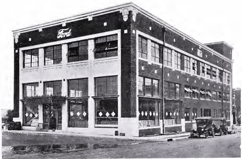
Fig. 12. Ford Agency for R. P. Rice, Kansas City, Kan. Smith, Rea & Lovitt, Architects
