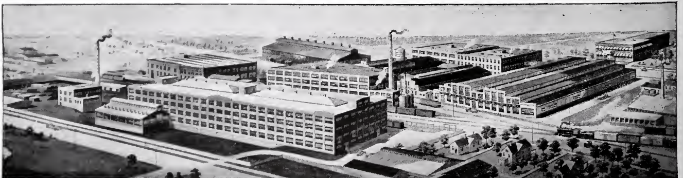
THE HAYNES AUTOMOBILE PLANT KOKOMO IND. Eight course built up Feltex over concrete
