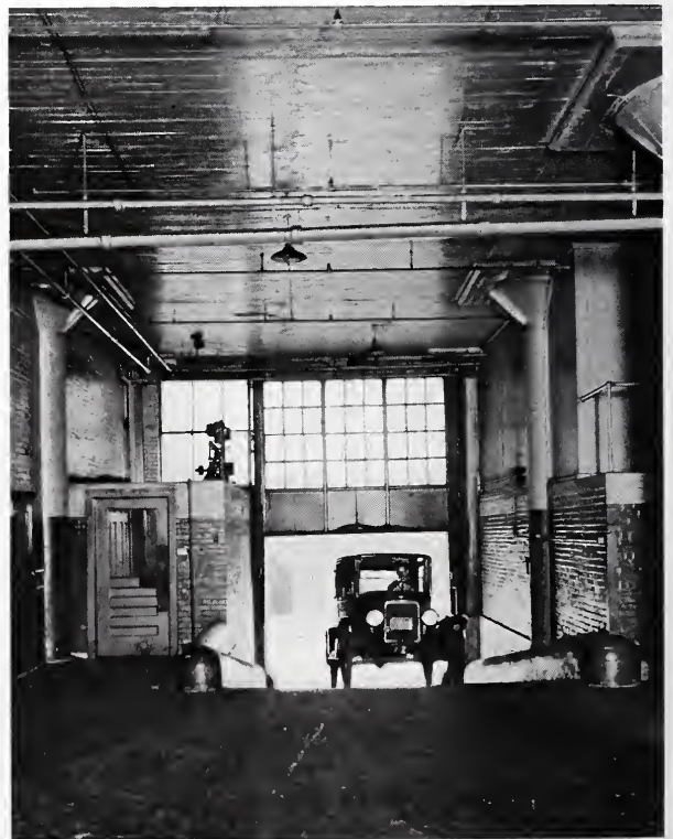
Entrance Ramp in Overland Building
