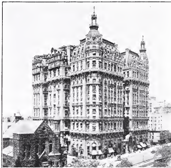
Hotel Ansonia, New York City: Warren & Wetmore, Architects; E. Smolka Plumbing Supply Co., Jobbers; James McCullagh, Plumber
