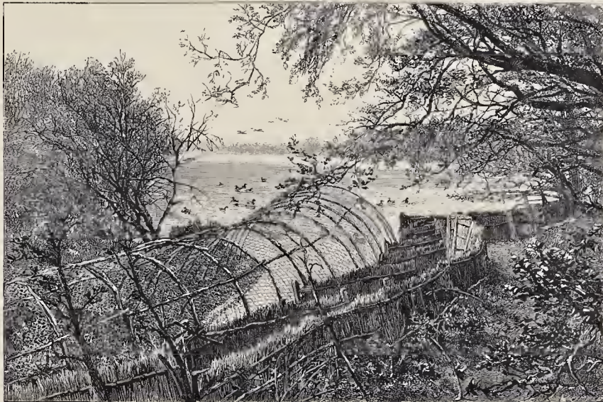
Outside the Pipe, looking towards Entrance.
