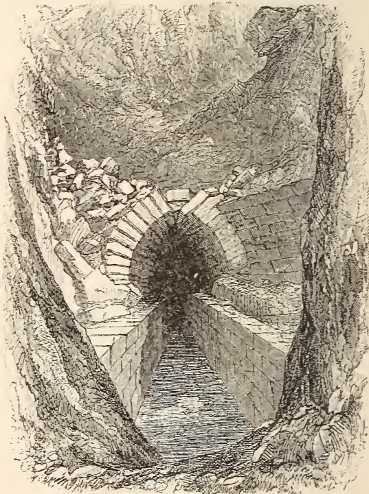
Vaulted Drain beneath the Palace at Nimroud. (From Layard's 'Nineveh'.)
