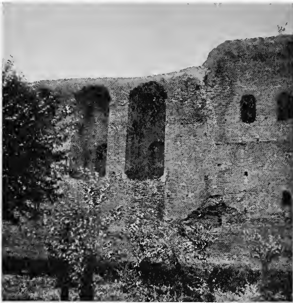
FIG. 14.— THE WALL OF AURELIAN, NEAR THE SESSORIUM.
