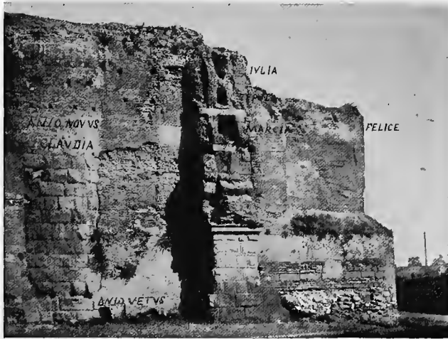
FIG. 10.—THE JUNCTION OF SEVEN AQUEDUCTS AT THE PORTA PRAENESTINA.
