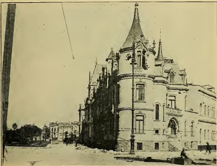
Windows on third floor shattered by shell from Arsenal
