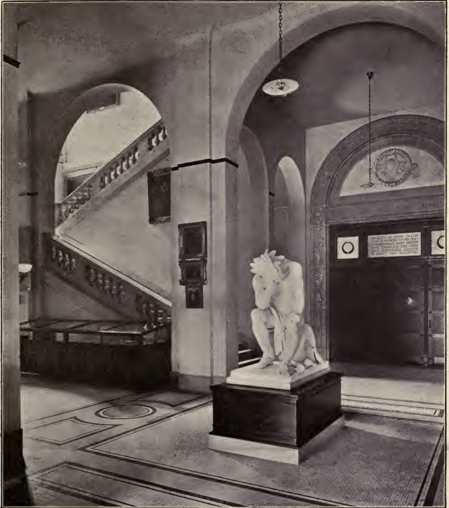
ENTRANCE HALL SHOWING STAIRCASE LEADING TO THE LIBRARY
