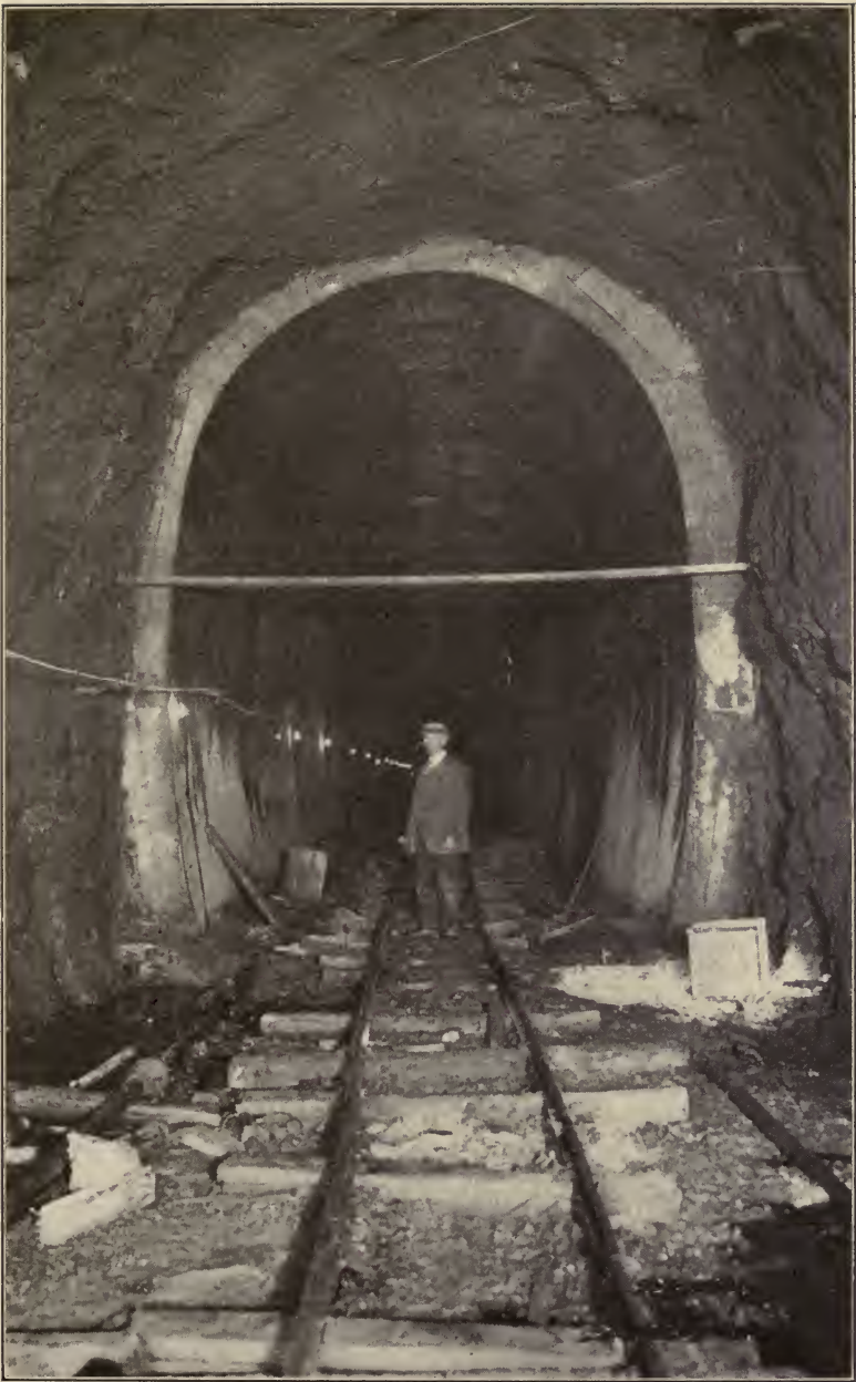
Bonticou Grade Tunnel, 17 feet high, 13 feet four inches wide, typical of other grade tunnel work
