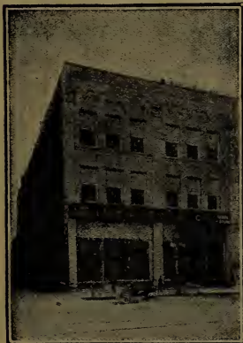
RETAIL STORE AND OFFICE 209-211 WALNUT STREET.
