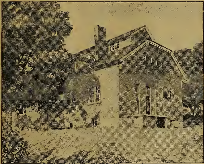
Front view of the storage-building
