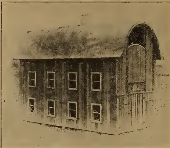
The barn as built for Kentucky conditions
