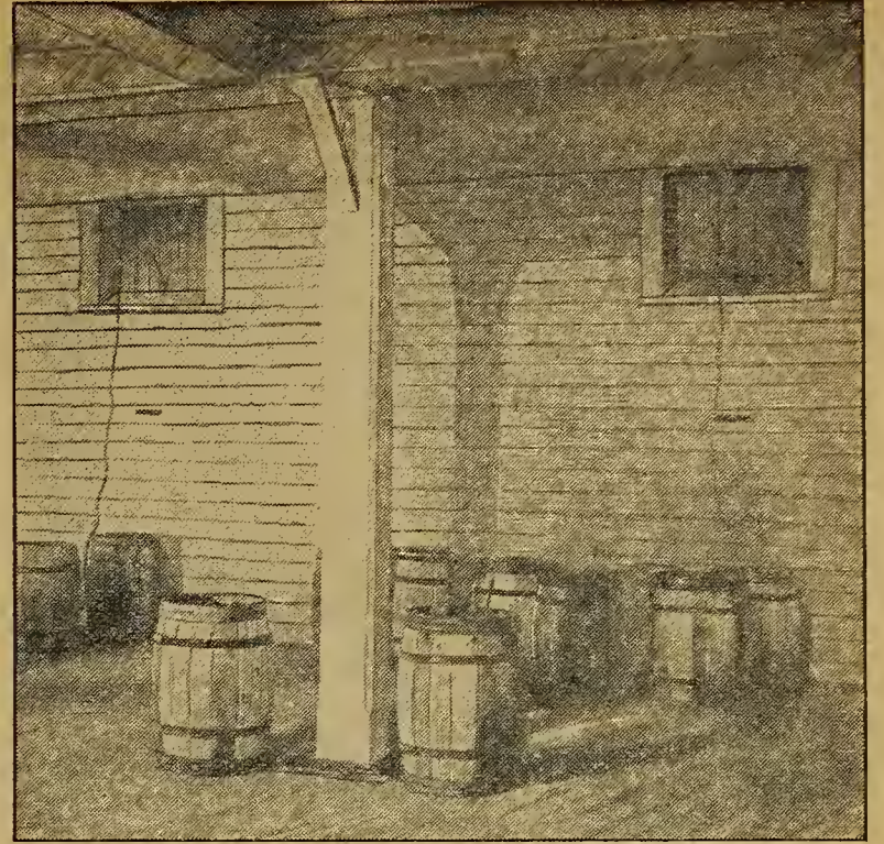
The frost-proof room in the basement. Windows, closed by shutters, are used for ventilation and cooling
