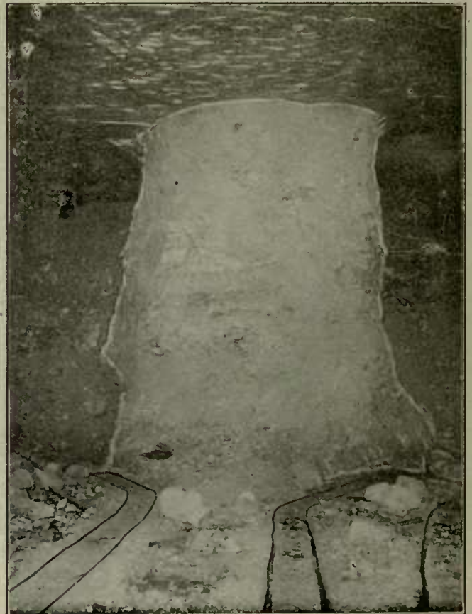
FIG. 11. CUTTING AROUND A PILLAR FROM TWO STOPS
