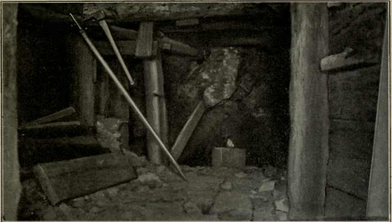
FIG. 23. TWO 16-FT. SPLICED STULLS FOR THE NEXT SET AHEAD IN THE CAVED PORTION OF A STOPE ARE TEMPORARILY SUPPORTED ON STRINGERS EXTENDED FROM UNDER THE CAPS OF THE SETS IN PLACE
