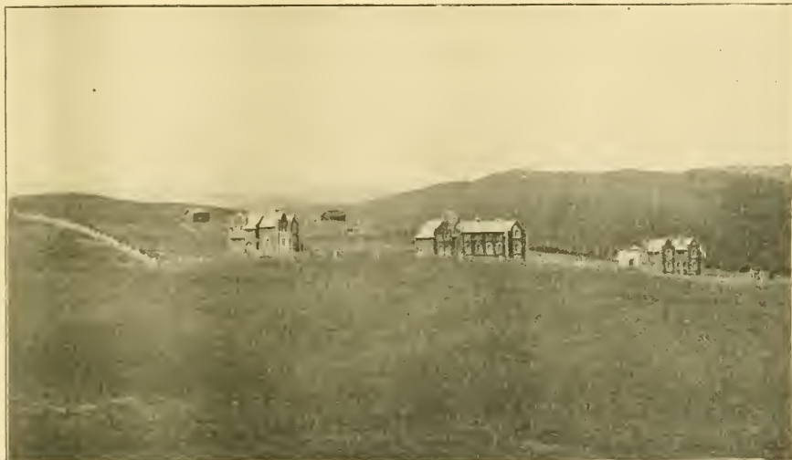
FIG. 3.—Eskdalemuir Observatory.—General view from the south-west. The office block is the middle one of the three buildings in line; the superintendent's house is on the left, the caretaker's house with assistants' quarters on the right. The two huts in the background are the wooden magnetic huts for "absolute" observations. In front of the right-hand hut is seen the mound of the underground magnetic chamber, with the stonework of the top of the porch. From the "Sixth Annual Report of the Meteorological Committee."
