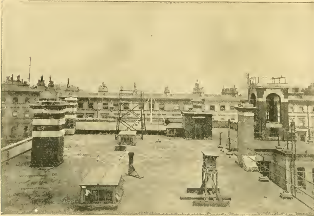
FIG. 1.—Meteorological Office.—Roof. From the "Sixth Annual Report of the Meteorological Committee," by permission of the Controller of H.M. Stationery Office.
