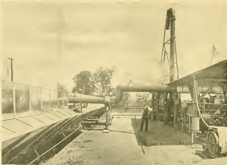
FIG. 1.—Showing one section of absorber on left, steam main and safety valve in centre, and part of engine on right
