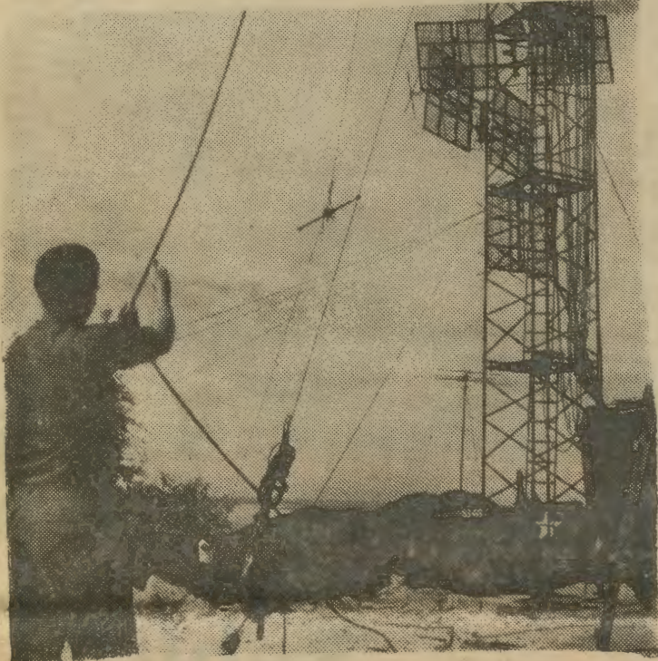
VC HILL ANTENNA — An unidentified member of the 518th Signal Company prepares to remove part of a "bedspring" antenna from a VHF antenna atop VC Hill, overlooking Vung Tau. Part of the 39th Signal Battalion, the 518th operates signal sites from Can Tho in the Mekong Delta north to Vung Chua Mountain, near Qui Nhon.
