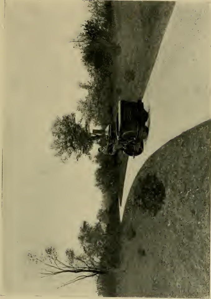
FIG. 16.—Park Walk. Drainage in Grass Gutters. Rolling being Done by Special Tandem Roller.
