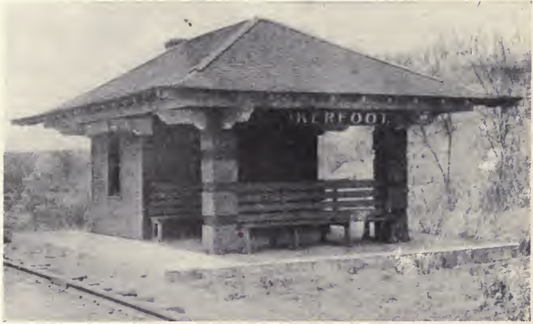
Fig. 152. Shelter Station, Ill. Traction System.
