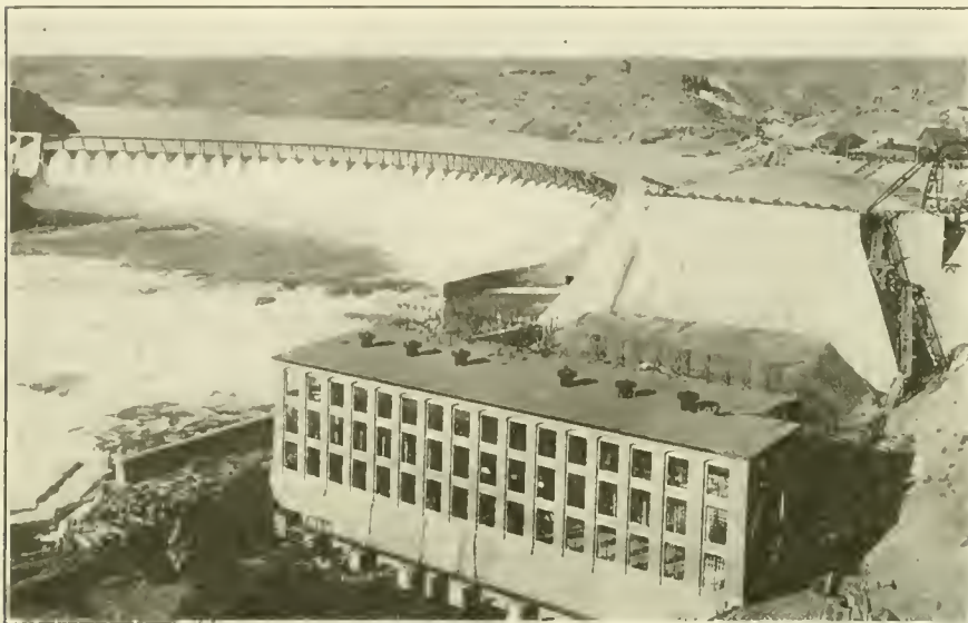
GENERAL VIEW GREAT FALLS DAM AND POWER HOUSE AT VOLTA, 4-10,000 K. W. VERTICAL GENERATORS FEED.
