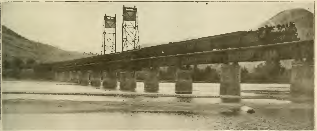
SINGLE LOCOMOTIVE HAULING FIFTEEN COACHES ACROSS THE THOMSON RIVER AND OVER THE ROCKY MOUNTAINS, BREAKING THE RAILWAY RECORD IN AMERICA. WEST BOUND GRADE 26 FEET TO THE MILE. EAST BOUND GRADE 37 FEET TO THE MILE.
