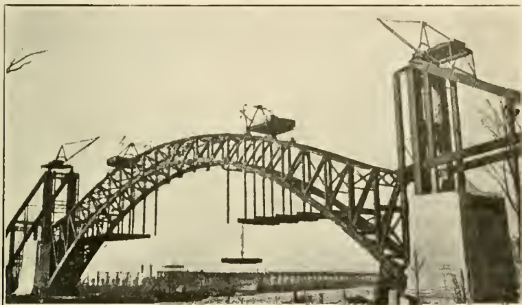
HOISTING A FLOOR BEAM ON THE HELL GATE BRIDGE.
