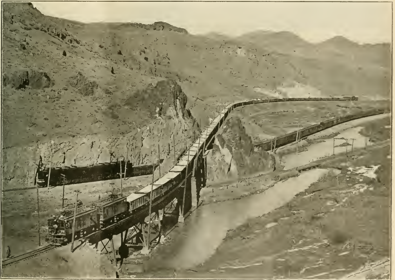
ORE TRAIN ON THE BUTTE, ANACONDA AND PACIFIC RAILWAY HAULED BY 2 80 TON 2,400 V. D. C. LOCOMOTIVES, AND FREIGHT TRAIN ON THE CHICAGO, MILWAUKEE AND ST. PAUL RAILWAY HAULED BY 3,000 V. D. C. LOCOMOTIVE
