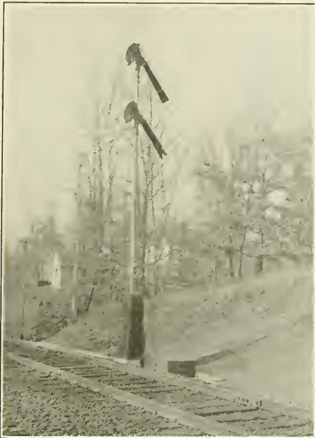
D. L. & W. SIGNALS OPERATED ON THE PERMISSIVE PLAN.
