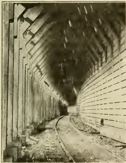
INTERIOR OF SNOW SHED ON THE CANADIAN PACIFIC RAILWAY.
