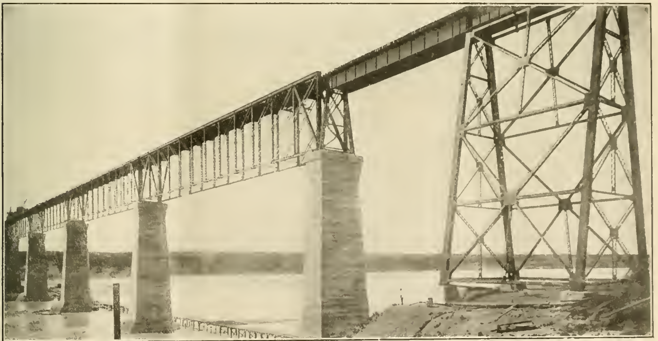
VIEW OF THE RIVER SECTION OF THE OUTLOOK BRIDGE AT LETHBRIDGE. AT THE RIGHT IS ONE OF THE NINE LAND TOWERS.
