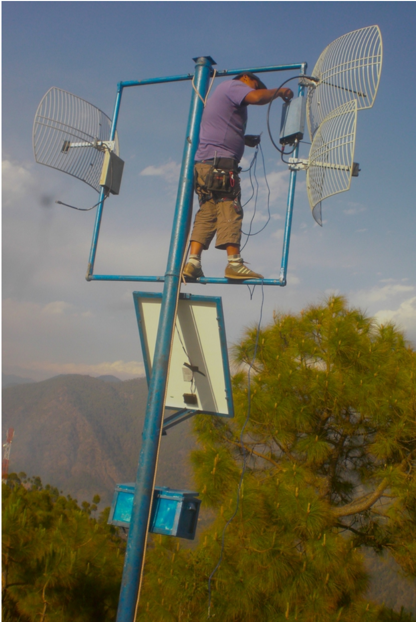
Figura EcA 8: Repetidora Troncal, Red de Garhwal
