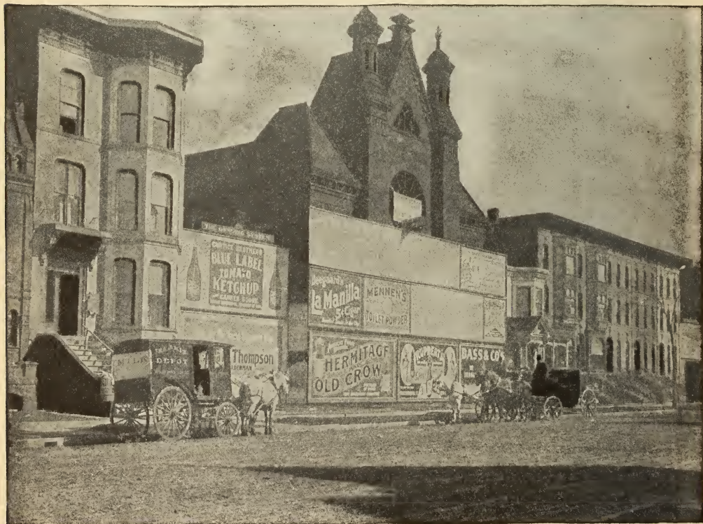
A thoroughly disreputable billboard, and a billboard which by frames is made fairly neat. The latter, however, is much too high—a "three decker"—and is out of place on its site.
