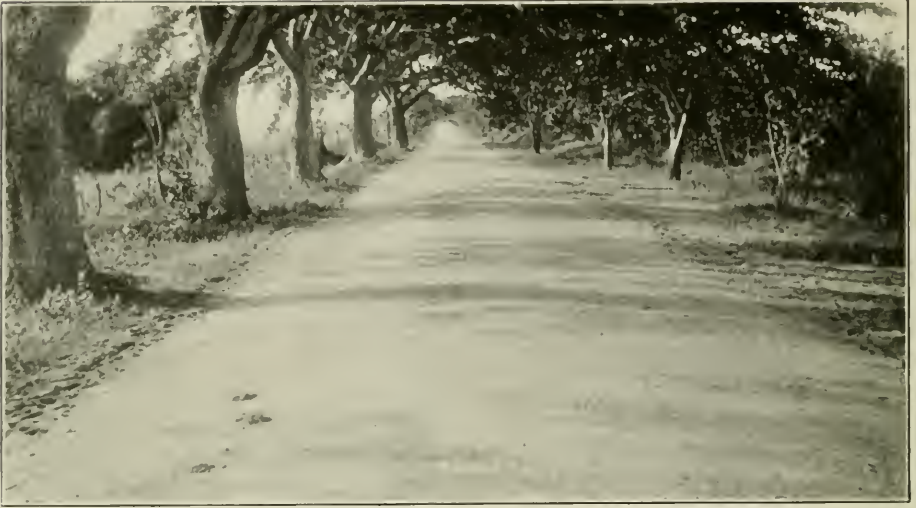
Road from Mariel after construction—Pinar del Rio Province
