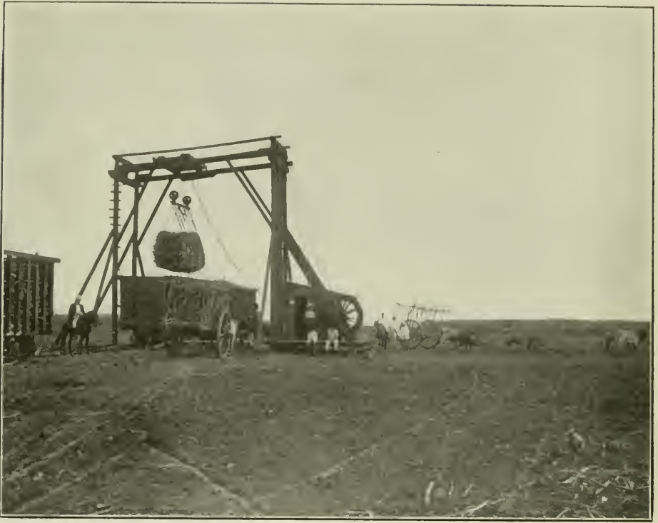
Handling cane by derrick from carts to cars.
