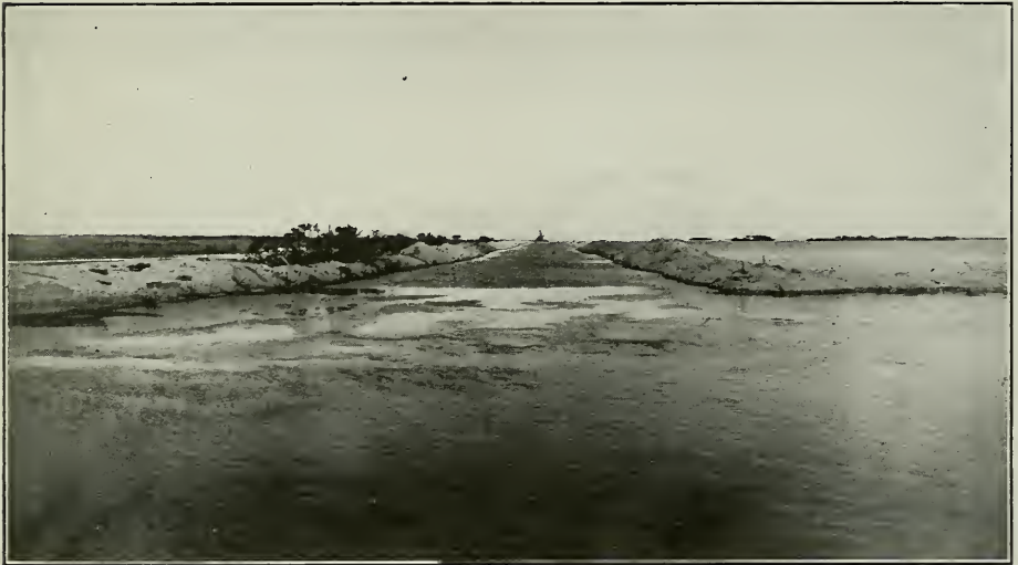
View of Canal which is being opened in Sabinal Bay—Camaguey Province.
