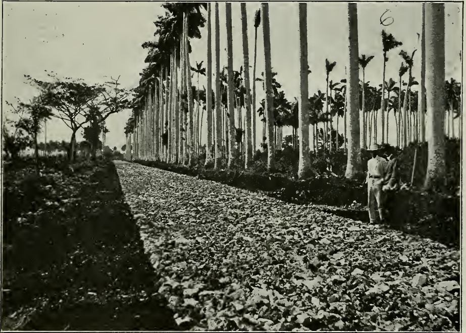
Road from Artemisa to the Cemetery under construction—Pinar del Rio Province.
