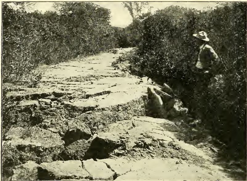
FIG. 3.—Road crossing the fault-line two miles southeast of Portola. There is a vertical uplift on the northeast side of the fracture at this place.
