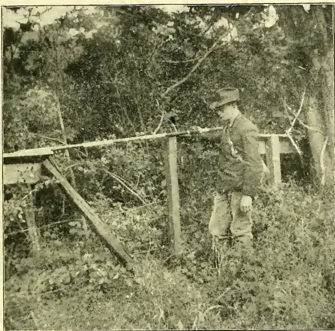
FIG. 4.—Showing a fence that crossed the fault at an oblique angle. The post shown in the photograph was split and pulled apart and the wires broken.
