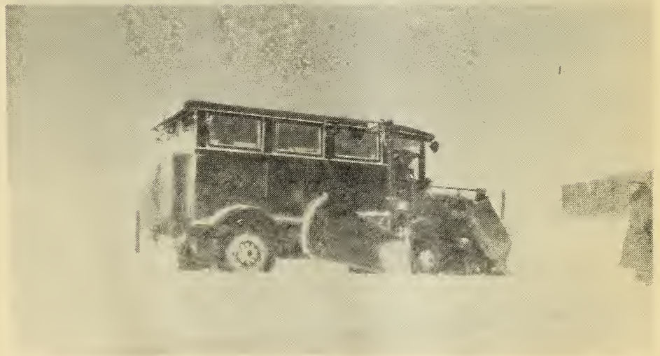
Figure 5--(above)--Twin motor trucks with V-plow used by the State of Minnesota.
