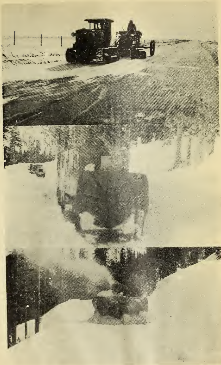
Figure 3--(above)--A representative snow-removal unit used by the Colorado State Highway Department.
