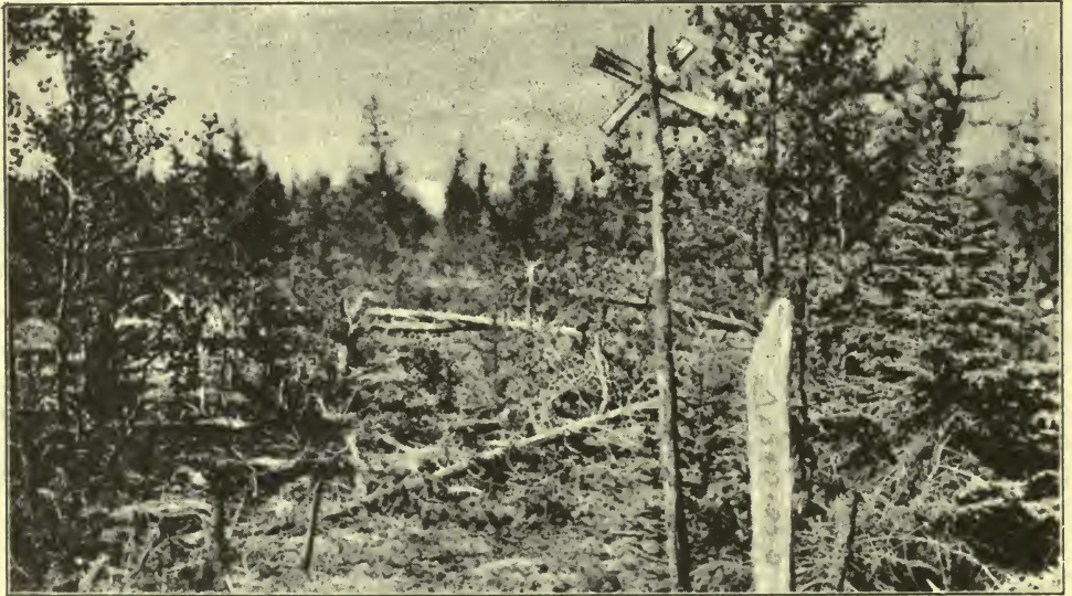
Typical Country on Hudson Bay Railway Survey.
