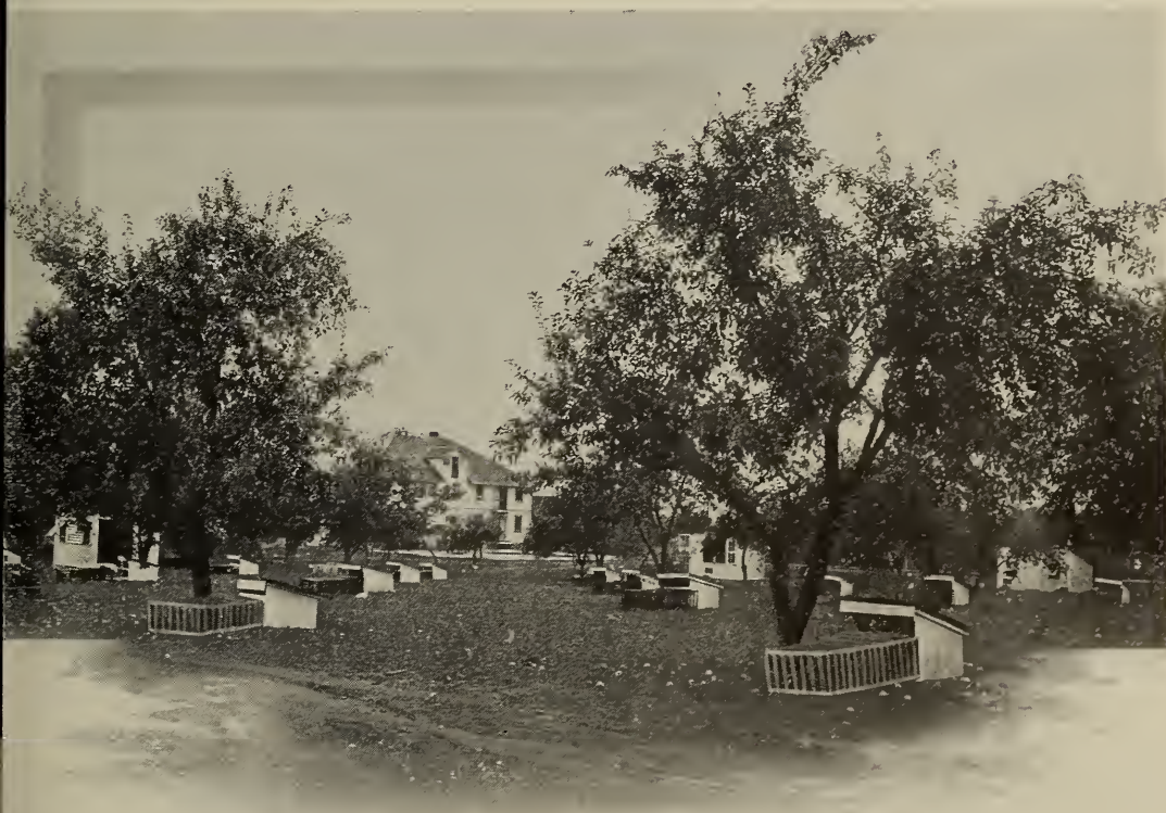
A view at the rear of the Administration building.
