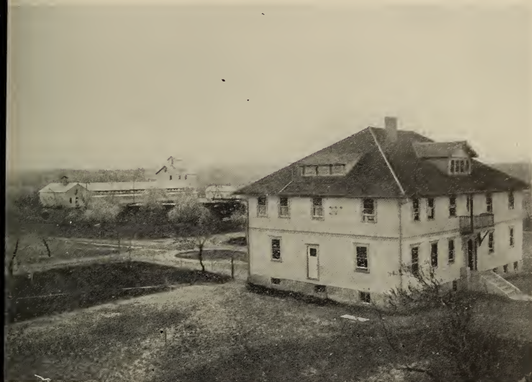
Administration building, brooder house, elevator, walks and driveways.
