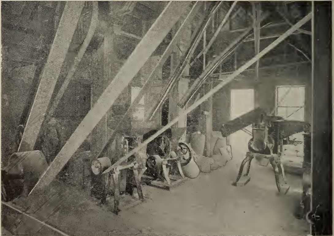
Interior of elevator and feed house—Shows a portion of machinery used in preparation and mixing feeds.
