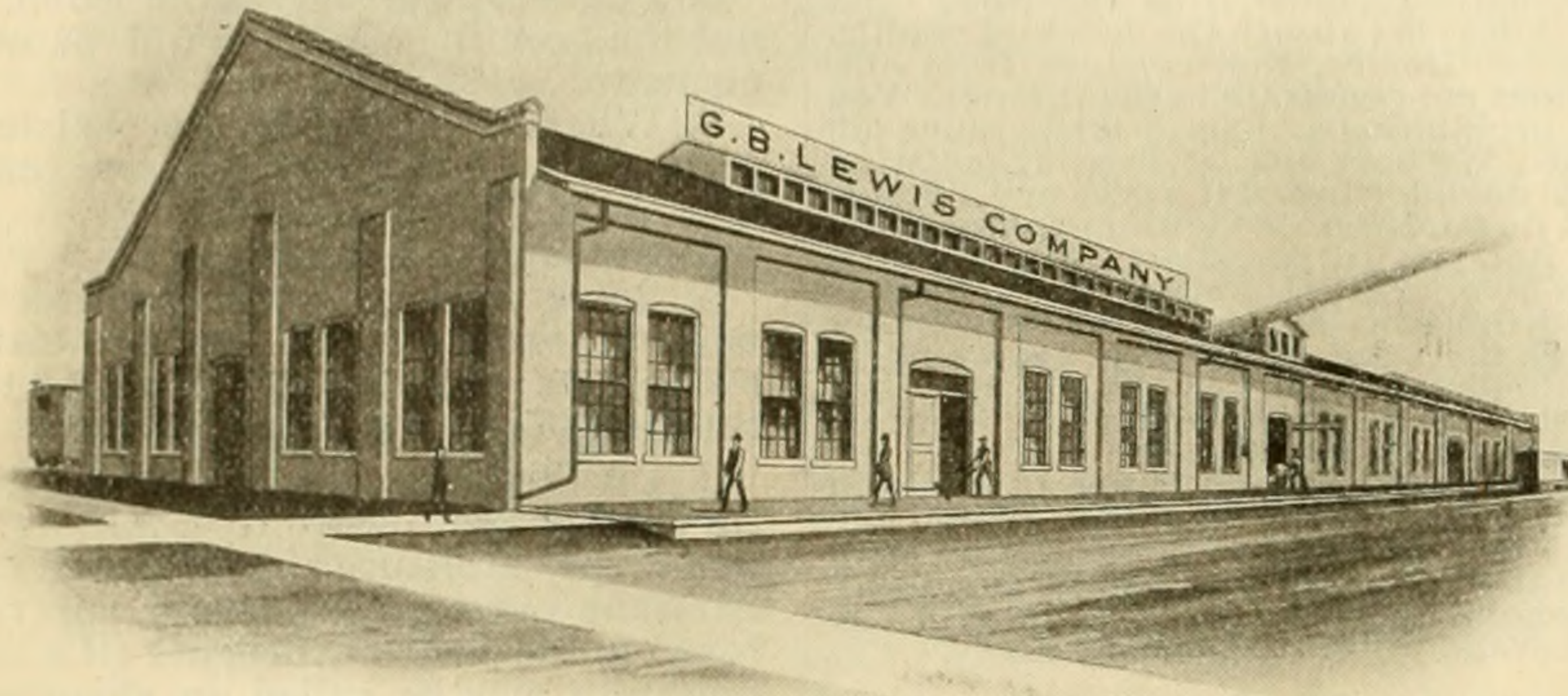
FIG. 1.—MAIN OPERATING PLANT OF G. B. LEWIS COMPANY, WATERTOWN, WIS.
