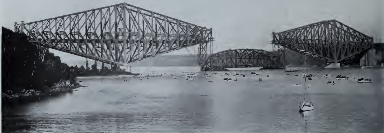
CENTRE SPAN MOORED AND READY TO BE LIFTED FROM PONTOONS.
