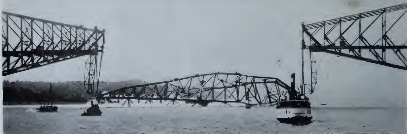
CENTRE SPAN COLLAPSING AND DISAPPEARING INTO RIVER AFTER HAVING BEEN LIFTED A FEW FEET. Copyrighted in Canada, Great Britain, and United States by Chesterfield & McLaren, Montreal.
