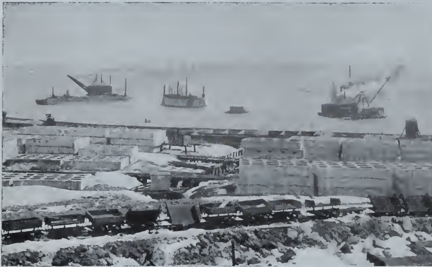
VIEW OF THE HARBOR—CELLULAR CONCRETE BLOCKS IN FOREGROUND.
