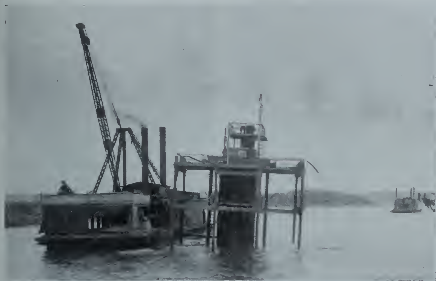
THE MOBILE PNEUMATIC CAISSON EMPLOYED.
