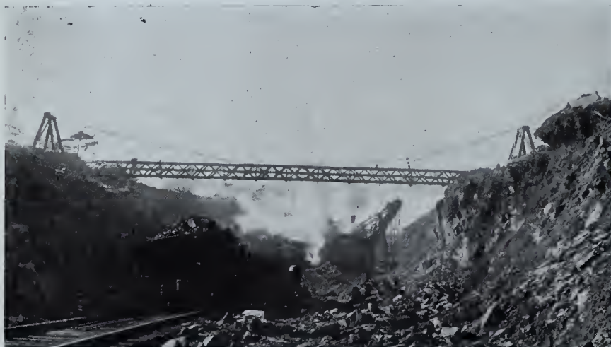
VIEW OF CUTTING SHOWING TEMPORARY BRIDGE FOR STREET.
