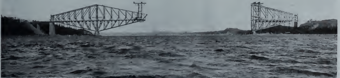
FIG. 4. GENERAL APPEARANCE OF BRIDGE AS COMPLETED UP TO NOVEMBER, 1915.
