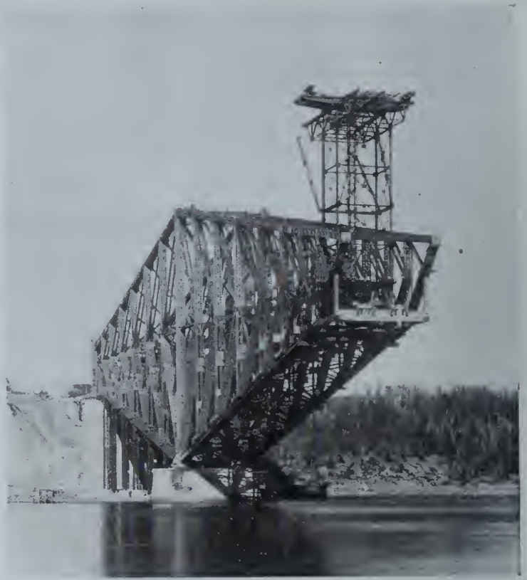
FIG. 5 NORTH SHORE TRUSS AS IT APPEARED ON NOVEMBER 7, 1915.
