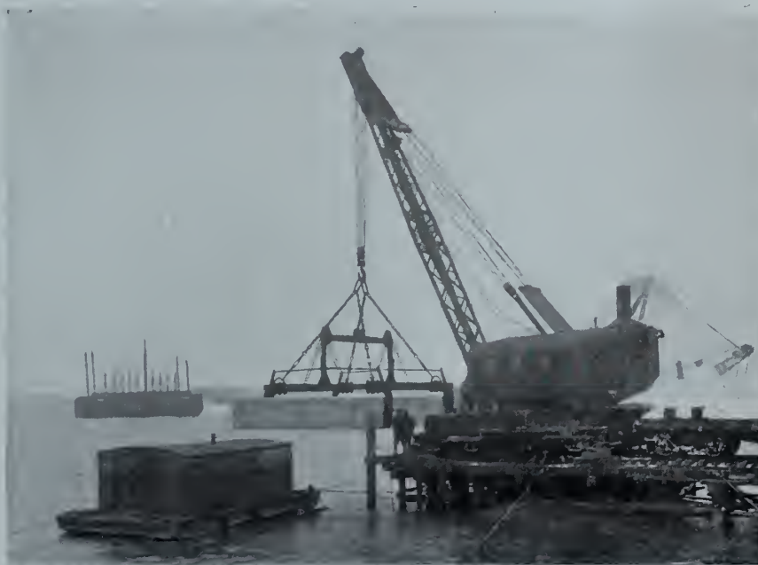
CELLULAR CONCRETE BLOCK BEING PLACED IN POSITION.
