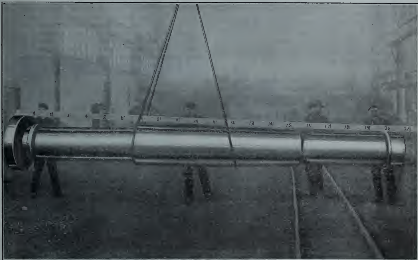
FINISHED COUPLING SHAFT, 18 IN. DIAMETER BY 21 FT. LONG
