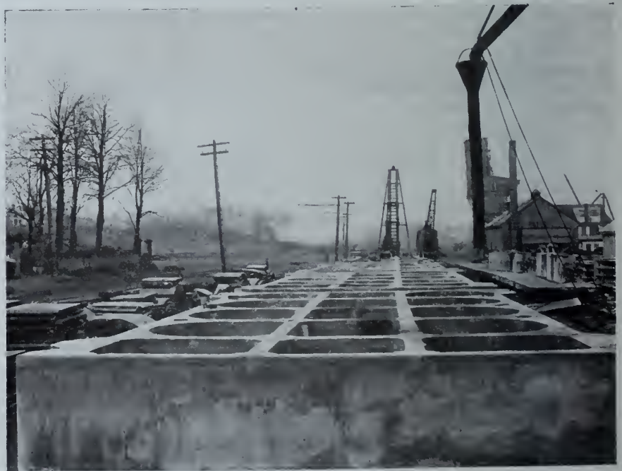
CLOSE VIEW OF THE CELLULAR REINFORCED CONCRETE BLOCKS.
