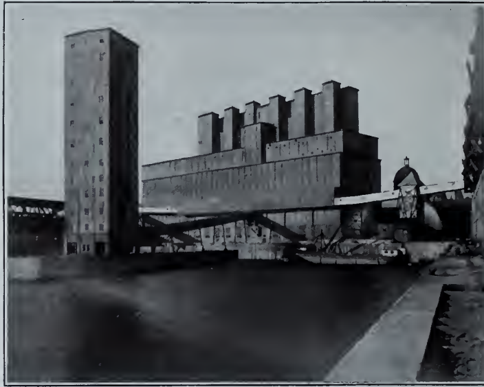
GRAIN ELEVATOR NO. 2 AND MARINE TOWER JETTY.
