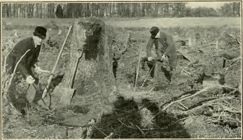
In blasting out big green stumps, the holes for the three to eight charges should be made as nearly as possible under the main anchor roots. The man on the right is smoothing out a hole, getting it ready for the charge; the one on the left is shoving a stick home with the tamping rod.
