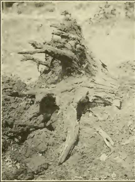
This stump came out as a result of a charge that was placed too deep and a little to one side of the proper position, and is not broken up for handling. It can be broken very easily as it lays, by locating a one stick mudcap charge between the two large roots seen in the picture. Had the original charge been a foot nearer the surface, the stump would have been broken in several pieces and all thrown out.
