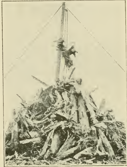
A type of "gin-pole" used to pile stumps for burning. Often piling by hand in small piles is much cheaper.
