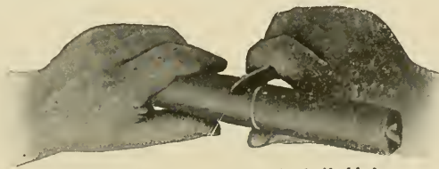
Cutting stick in two—roll it under knife blade
