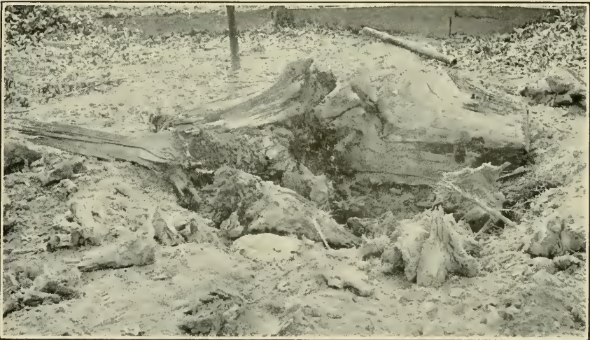
As these roots lie, they show the result of an almost ideal blast. There is little hole in the ground; the stump is well broken up; the roots are cleaned of dirt; and no roots have been thrown very far.
