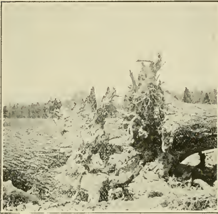
Two large hardwood trees which stood close together and were blasted out at one shot, without cutting down. About eight charges were used. The cavity in the ground is small and the soil is free from tight roots.
