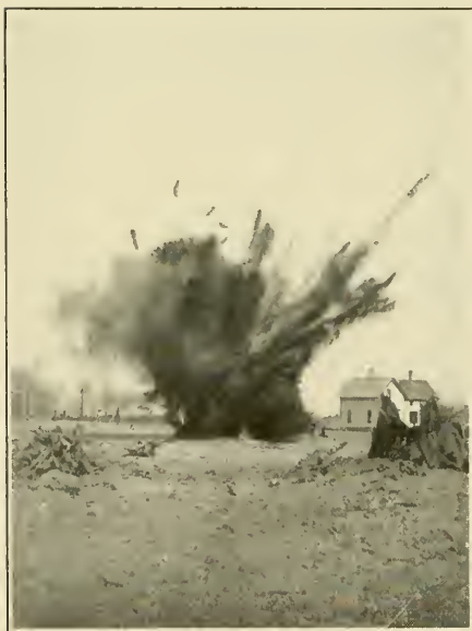
Some such appearance is necessary in stump blasting, but the less of it there is the better. The ideal blast is just strong enough, and is so located, that it rolls the roots free of their beds and splits them apart, but does not throw them an unnecessary foot. Loud reports and much dirt high in the air show careless loading and useless expense.
