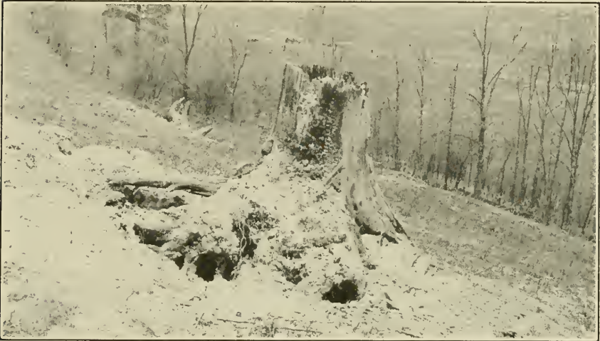
Four charges fired together tore this stump loose from its moorings and moved it six feet down the hill, but did not break it up. Another charge should have been located close under the center. It can be broken up easily now, however, by loading one stick charge down in the center of the hollow top. THIS STUMP IS A WHITE PINE, CUT 75 YEARS AGO.
