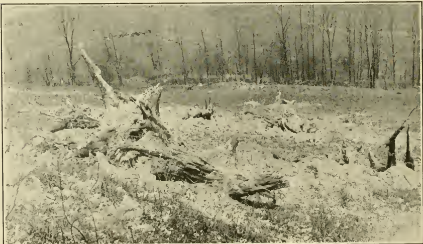
A very old white pine stump blown out with three charges fired together electrically. The stump is well torn loose and cleaned, but another charge should have been placed at a point close to the wood under the center, to split the stump for easy handling.
