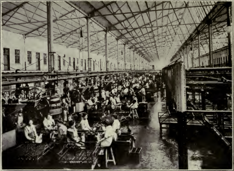
Interior from Carlsberg Bottlery, Copenhagen, Denmark.
