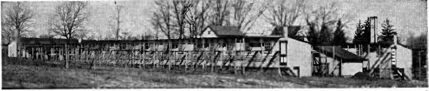
FIGURE 11.—Hip-roof house with closed front, used in New Jersey.
