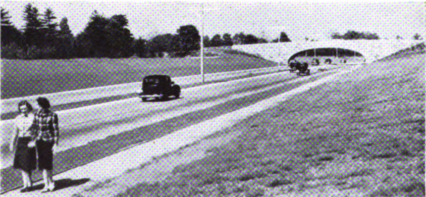
All rural sections of the system carrying traffic of 10,000 or more vehicles daily are located within zones of traffic influence of cities. The above view of Northern State Parkway at Westbury, Long Island, is fairly representative of the type of construction proposed. Costs may range from $150,000 to $700,000 per mile, depending largely upon right-of-way expense.
