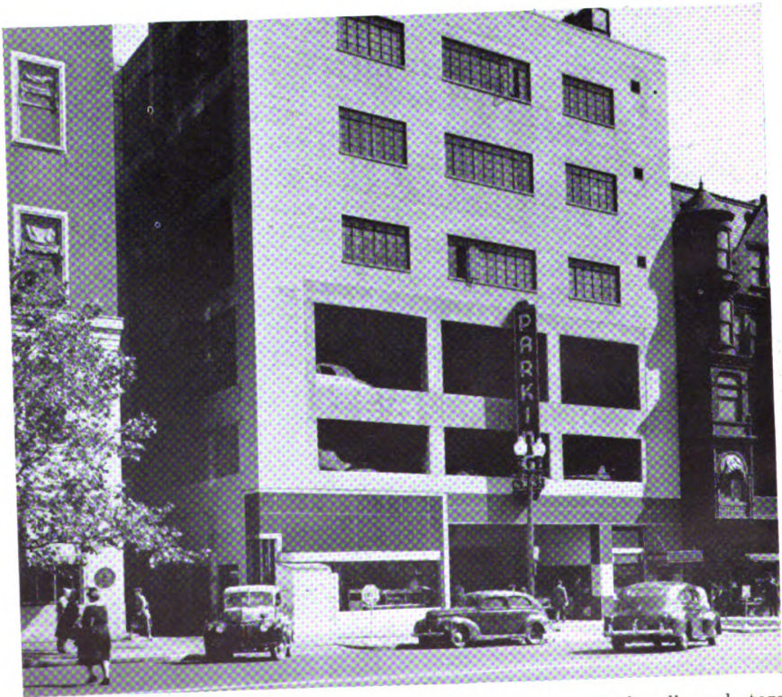
PLATE VI.—Examples of open-wall parking garages with grilled walls and store frontage (upper) and with upper stories devoted to office, loft, or other uses (lower). In this case the upper stories are occupied by bowling alleys. Such structures are suggested as the possible prototypes of a most desirable solution of the parking problem.
