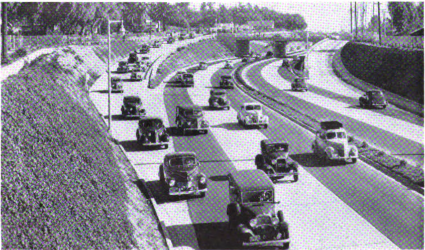
This example, like the one above, embodies many of the features considered desirable for urban depressed construction, but is also somewhat cramped in its design by inadequate right-of-way width.
