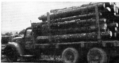
Figure 87.—Flat-bed truck with log-carrying bunks.
