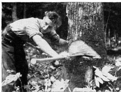
Figure 54. —Testing the undercut to make sure the tree will fall in the direction wanted. (Man should be wearing a hard hat.)
