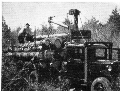
Figure 86.—A self-loading truck.
