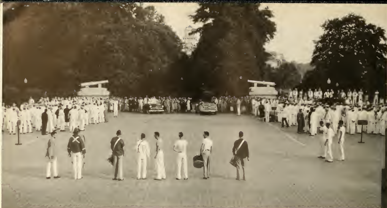
NO INSPECTION . . . NO INHIBITIONS.
