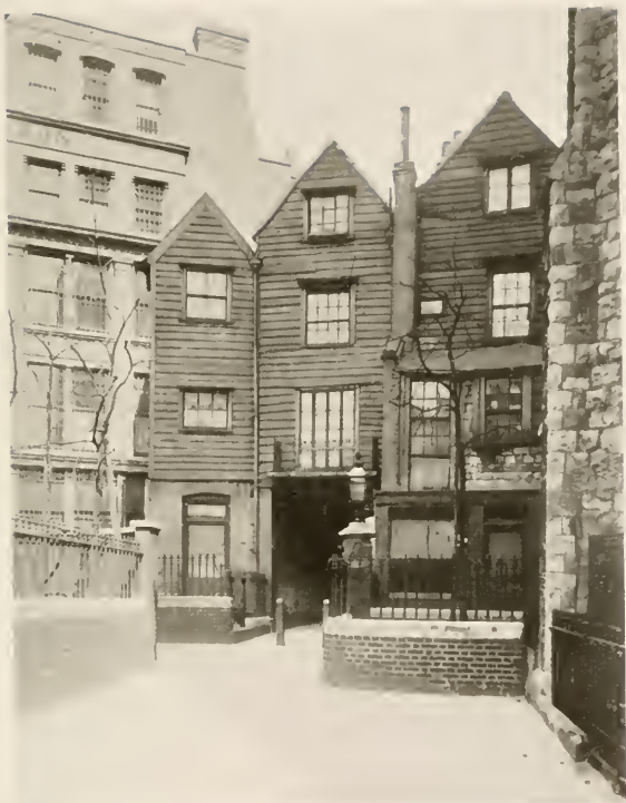
OLD WOODEN HOUSES AT CRIPPLEGATE (RECENTLY DEMOLISHED).
