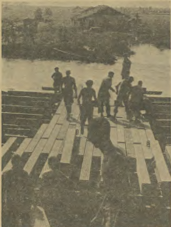
Men of the engineer battalion emplace sections of a bridge.
