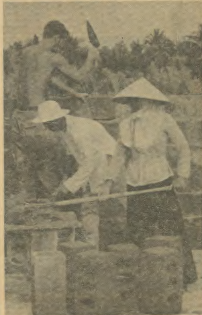
One man, employed by the engineers, became a bricklayer.
