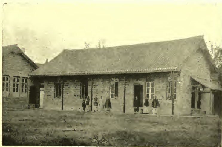
OUR FIRST HOSPITAL IN WEST CHINA.
