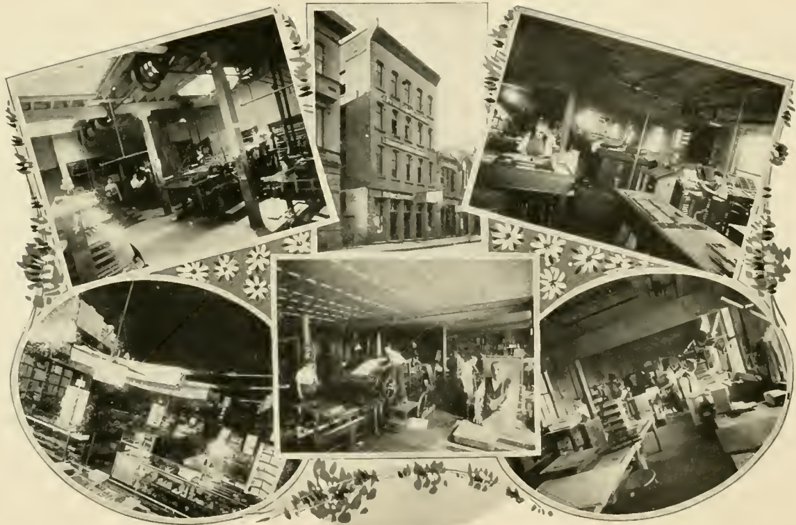
Corner of Cylinder Press Room Portion of Retail Store
