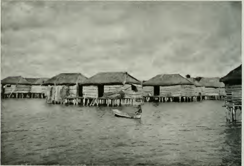
The pile-built villages in the lagoon of Sinimaica are survivals of the ancient villages of the Indians from which the name Venezuela—Little Venice—was derived. All traffic is by boat and you step from the wobbly dugout upon ladders rising from the water and find yourself on a shaky platform of small poles. Within the house you sit on your heels and eat toasted plantains and boiled manioc, while beneath you little scavenger fishes watch eagerly for crumbs that may fall through the latticed floor
