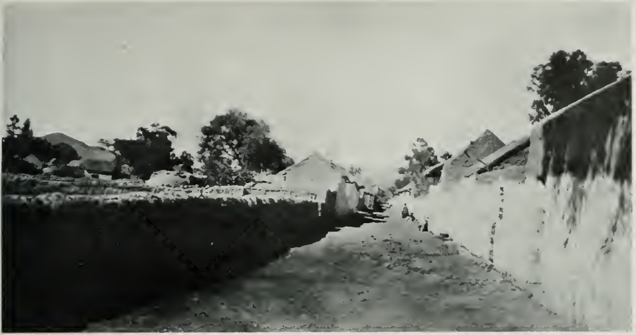
The Quichua Indian village of Puna is built entirely of adobe. It seems as if a heavy rain would wash all the structures away, but they are nevertheless able to withstand climatic conditions for a number of years
