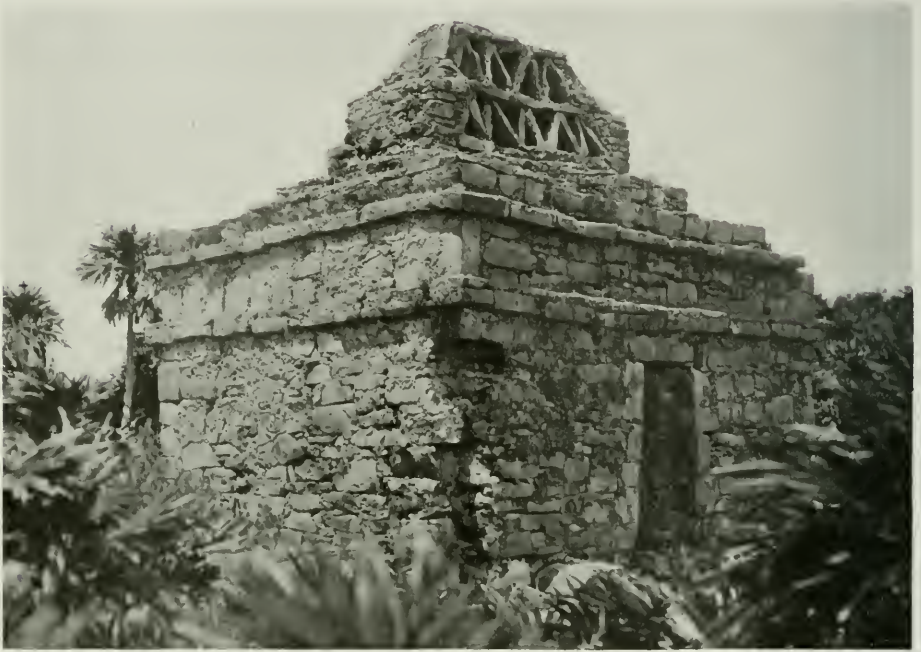
This small temple, standing a few hundred yards outside the walls to the north, presents a feature common in Maya architecture—namely, the roof comb, a wall purely decorative in purpose and usually embellished with an elaborate design in stucco
